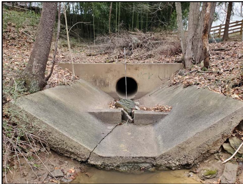
CA-5 Photo Point 101 36" Reinforced Concrete Pipe with Energy Dissipation into Tributary 1
