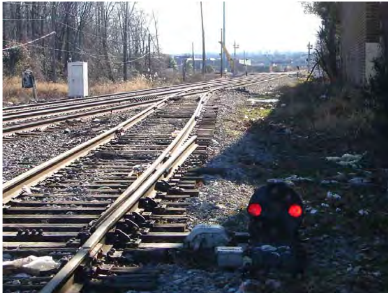
Historic Image 4: Signal (Circa 1920s) A B&O Color Position Light-Type Signal at MP#28 Photographed December 2014. From www.trainweb.org .
