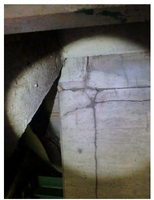
Photo 27: Seven Locks Road (106010) – looking at cracks in concrete support between inner and outer loops
