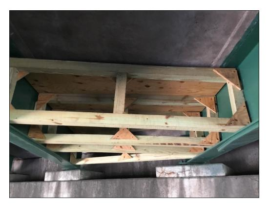
Photo 24: Greenbelt Road Outer Loop (141015) - Wooden braces obscure view of and access to the northwest abutment wall.
