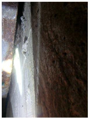
Photo 58: Cedar Lane (122010) – Looking at crack between abutment and deck on east abutment
