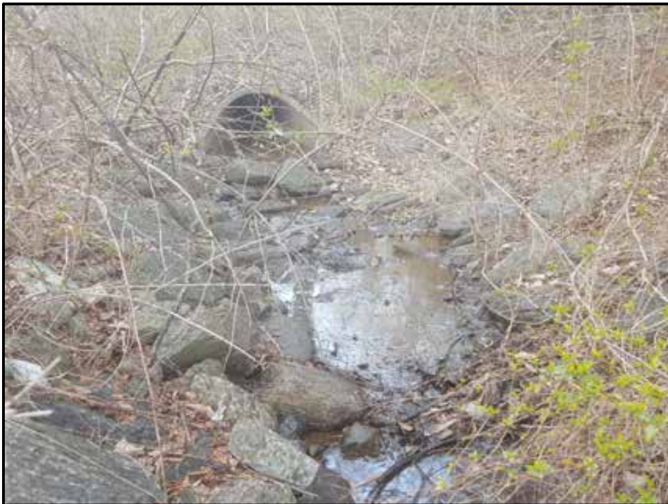
Waterway 27L – Intermittent
