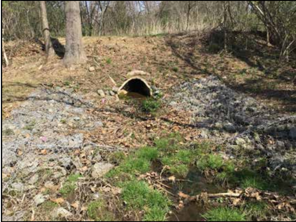
Waterway 26L – Intermittent
