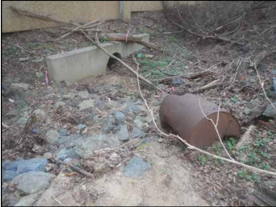
Waterway 21F – Intermittent
