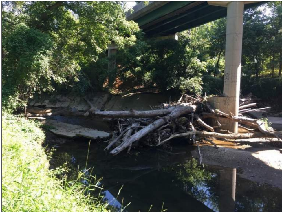
Figure 56. Concrete armoring on the Cabin John stream bank, with I-495 bridge visible in top right, facing northeast
