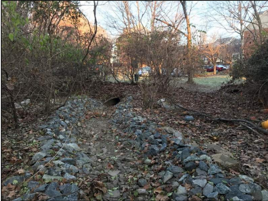
Figure 24. Improved rip-rap drainage feature in Area S-10, facing northeast
