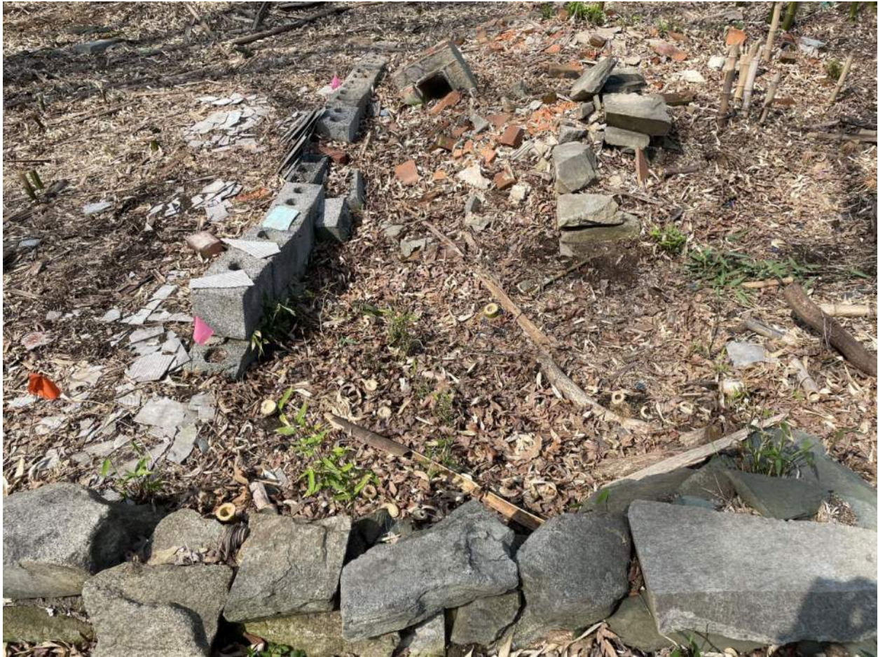
View west at the south end of the Moses Hall foundation showing concrete block, chimney remnants, and stone foundation wall.
