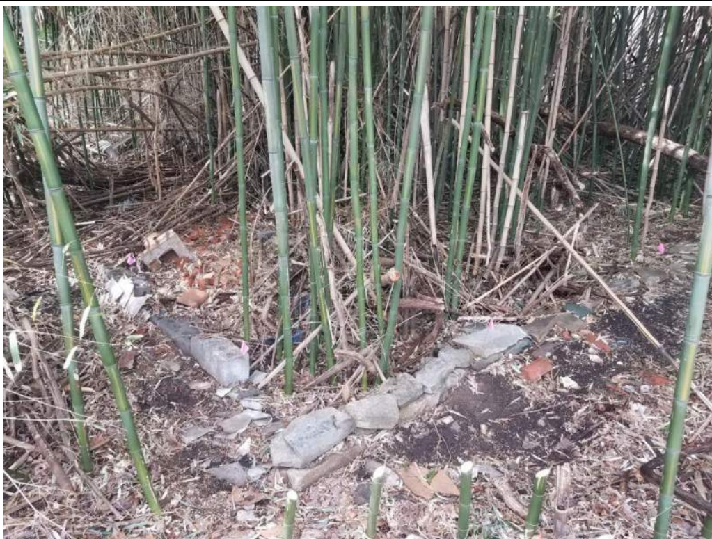
View of exposed SE corner of lodge foundation, east wall constructed of fieldstone, outside southern wall is concrete block, interior southern wall is fieldstone, looking northwest.
