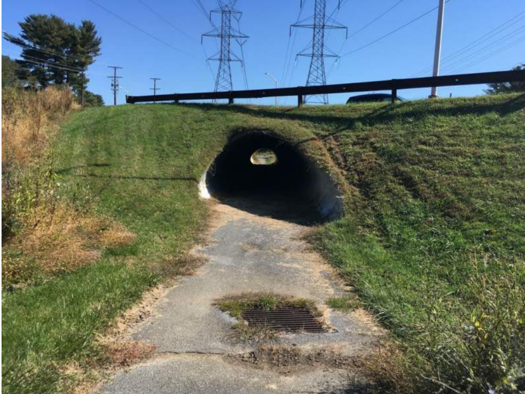
View facing west towards Montgomery Village Avenue, showing corrugated metal pipe tunnel allowing golf cart passage beneath the roadway.
