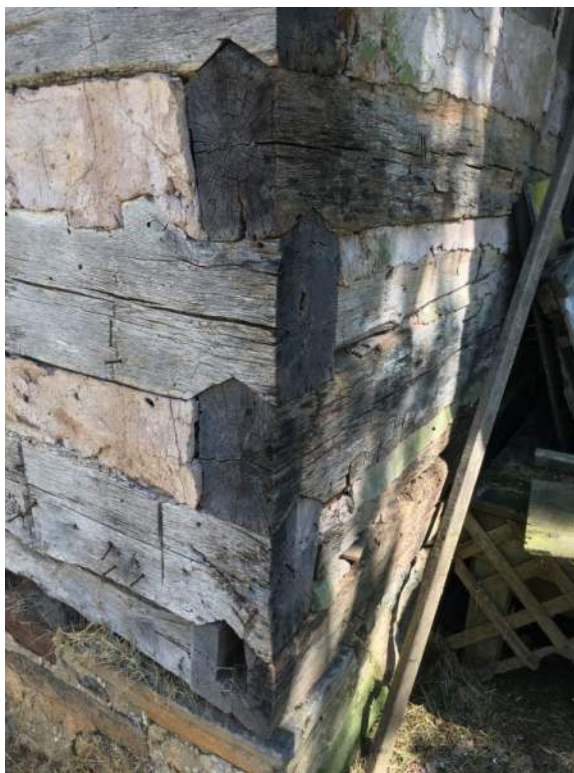
Detail showing V-notch timbering; southwest corner of log house
