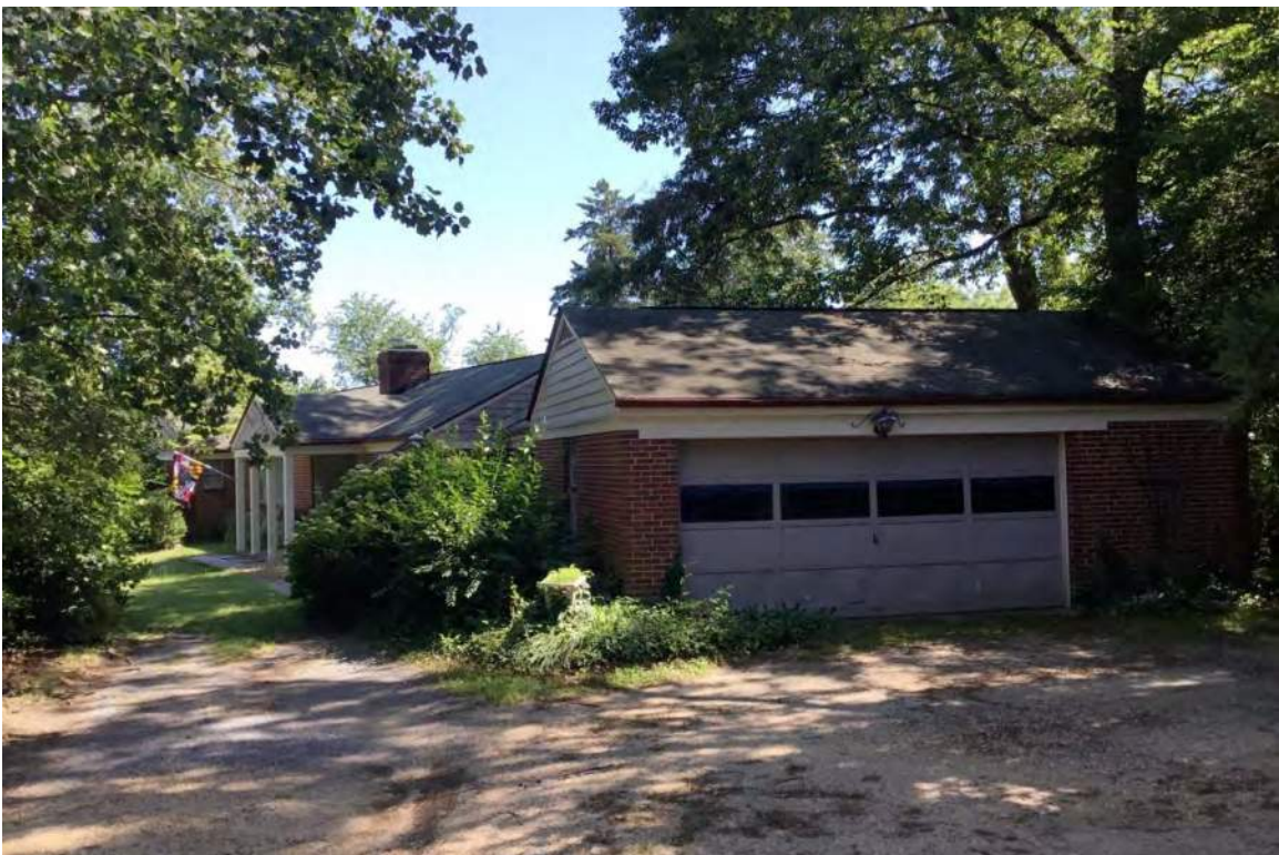
Northeast facade and garage north elevation
