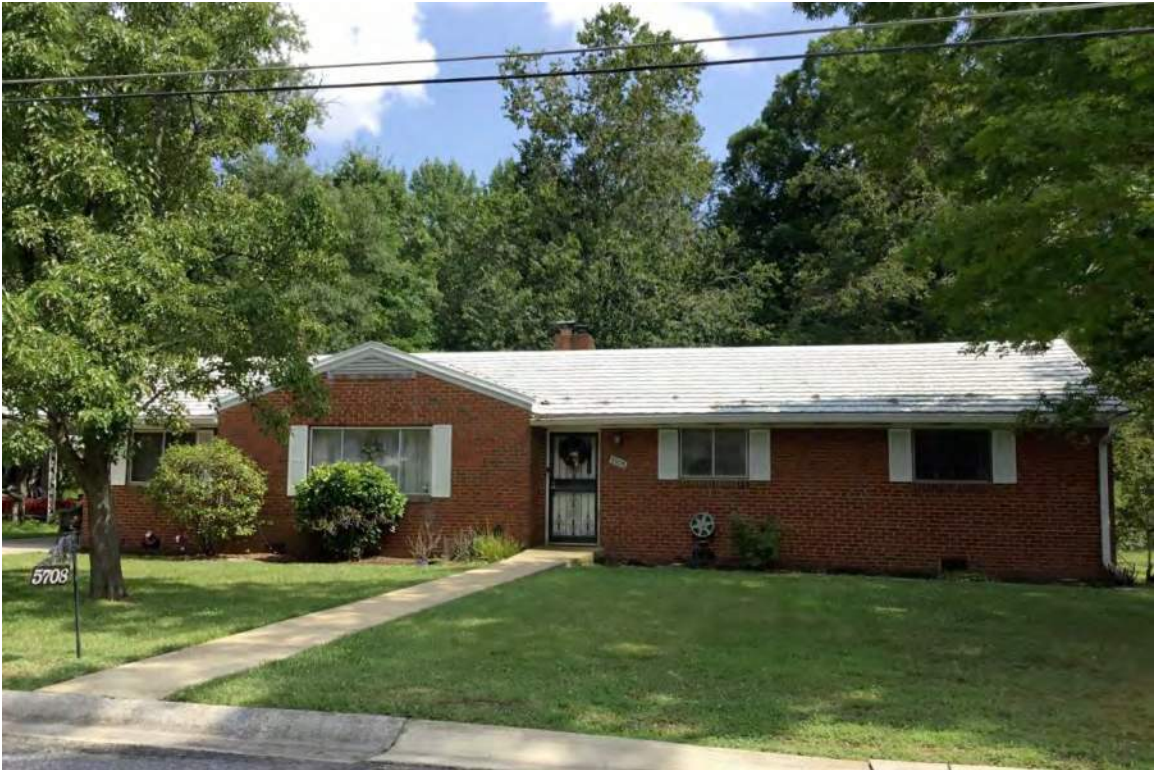
Primary elevation of 5708 Center Drive, looking south.
