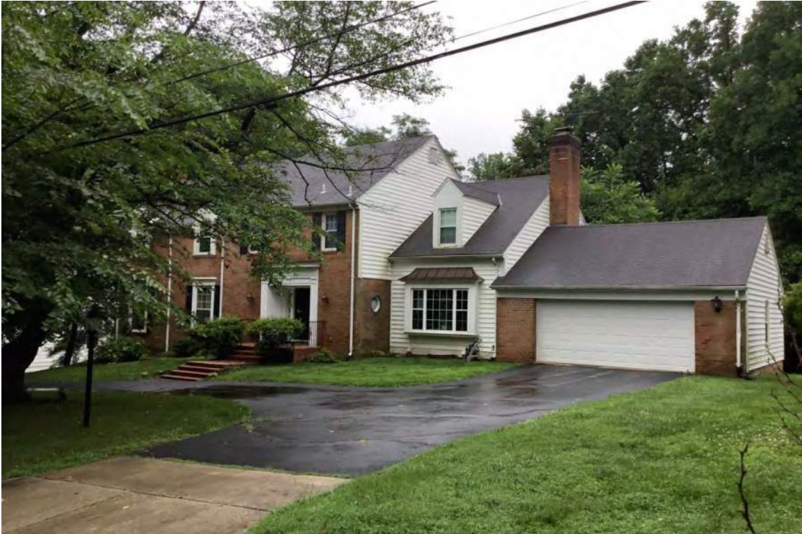
Oblique of 7100 Heatherhill Road, looking south.
