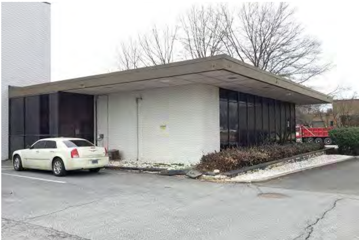
View facing southwest towards showroom.
