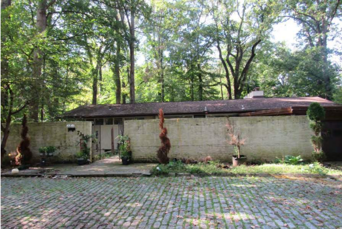
North elevation (façade)
