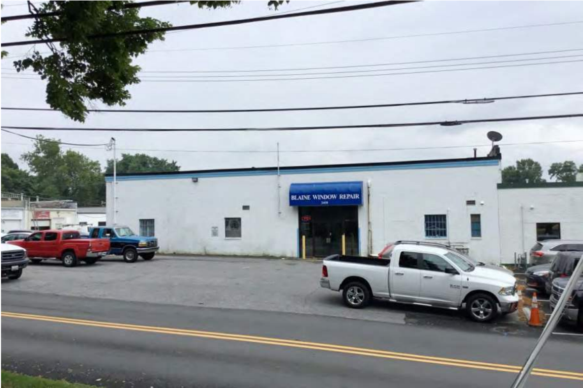
2410 Linden Ave, North Elevation Looking South
