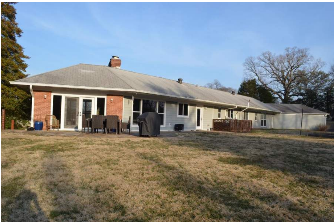
Dwelling, southwest elevation looking east
