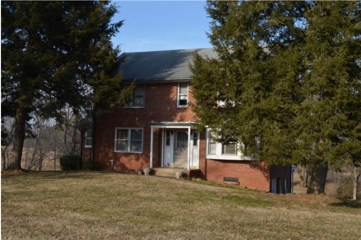
Dwelling, southwest elevation looking north
