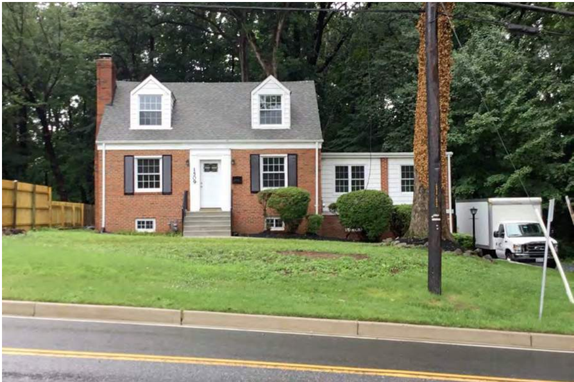
South elevation of 1509 Forest Glen Road.
