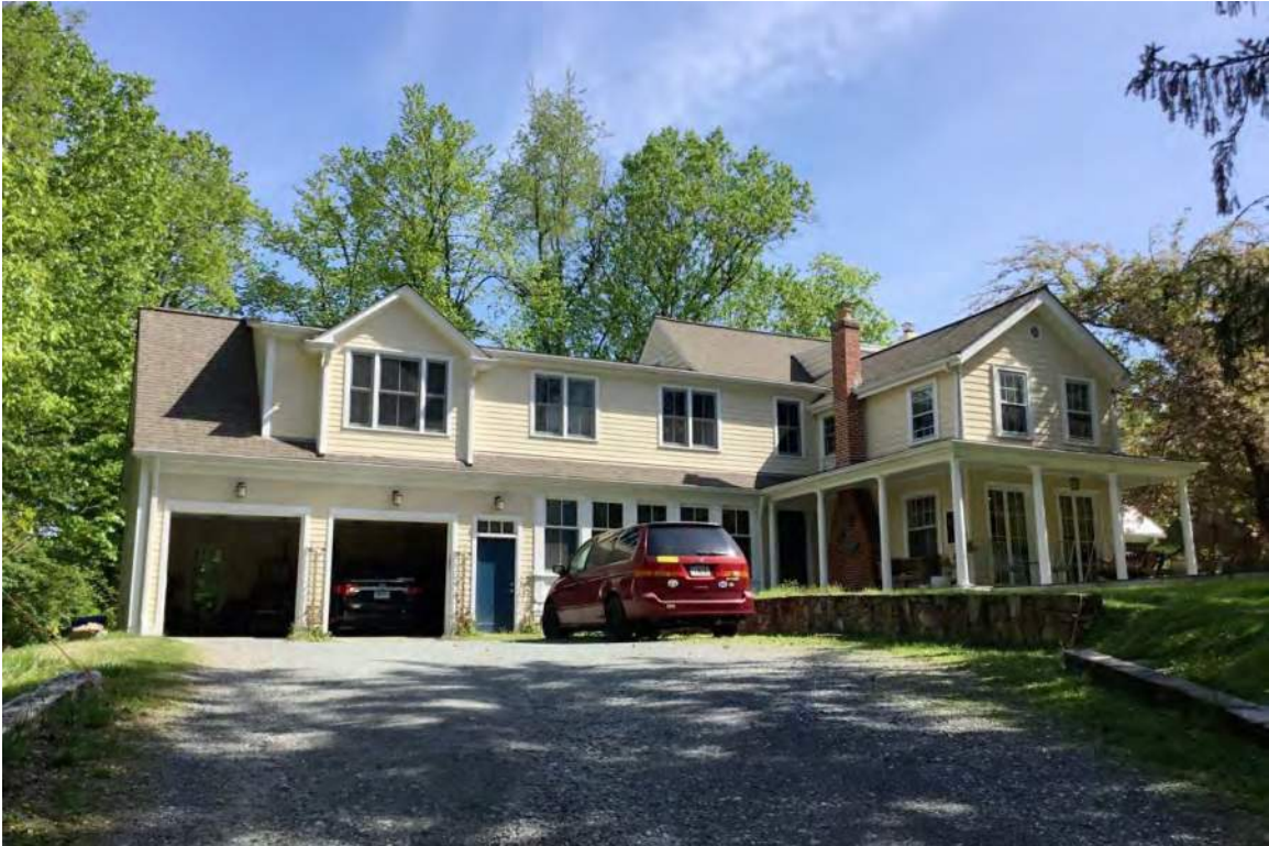
South elevation (façade) of 9017 Spring Hill Lane, looking north.
