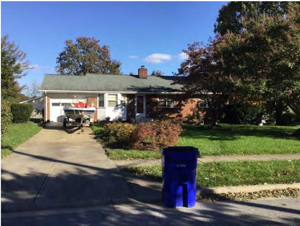
West elevation (façade) of 9907 51st Avenue, looking east.
