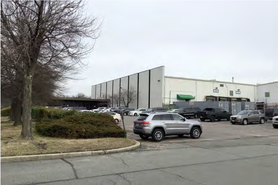
View facing northeast towards 3900 Penn Belt Place.
