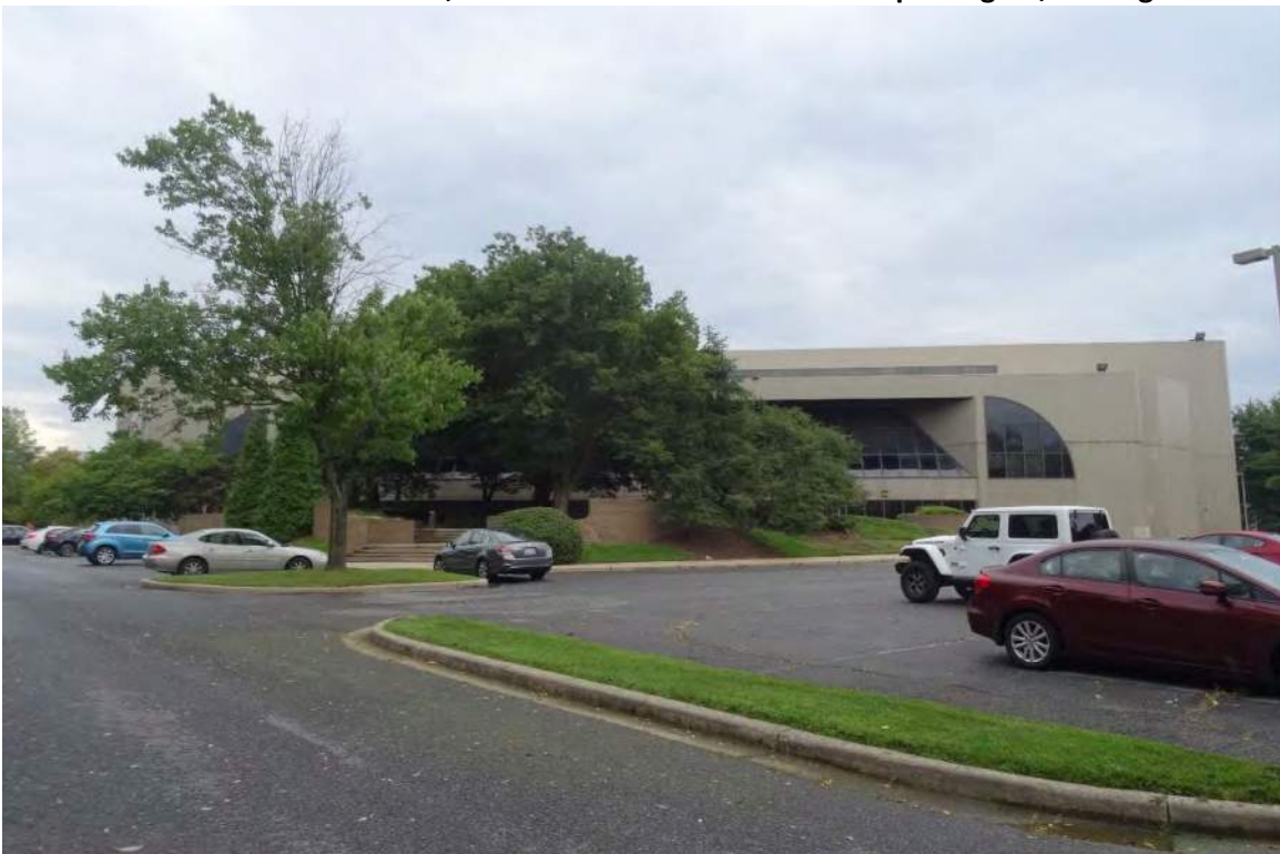
Photo 4 of 8: 1350 Piccard Drive, west elevation. View from parking lot, looking east.
