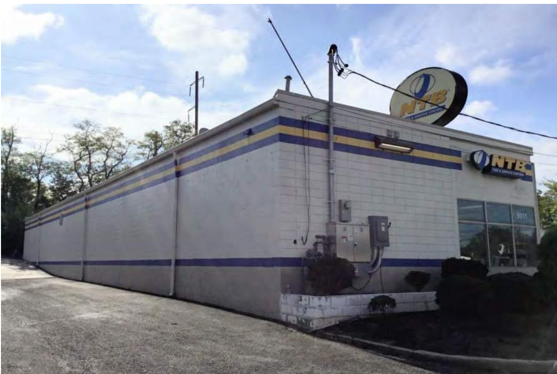
East oblique of 9011 Annapolis Road.
