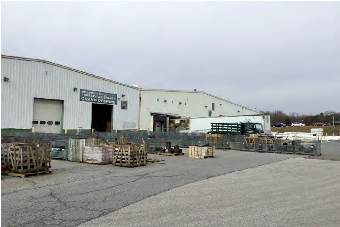
View facing west towards east east elevation of 3900 Penn Belt Place.
