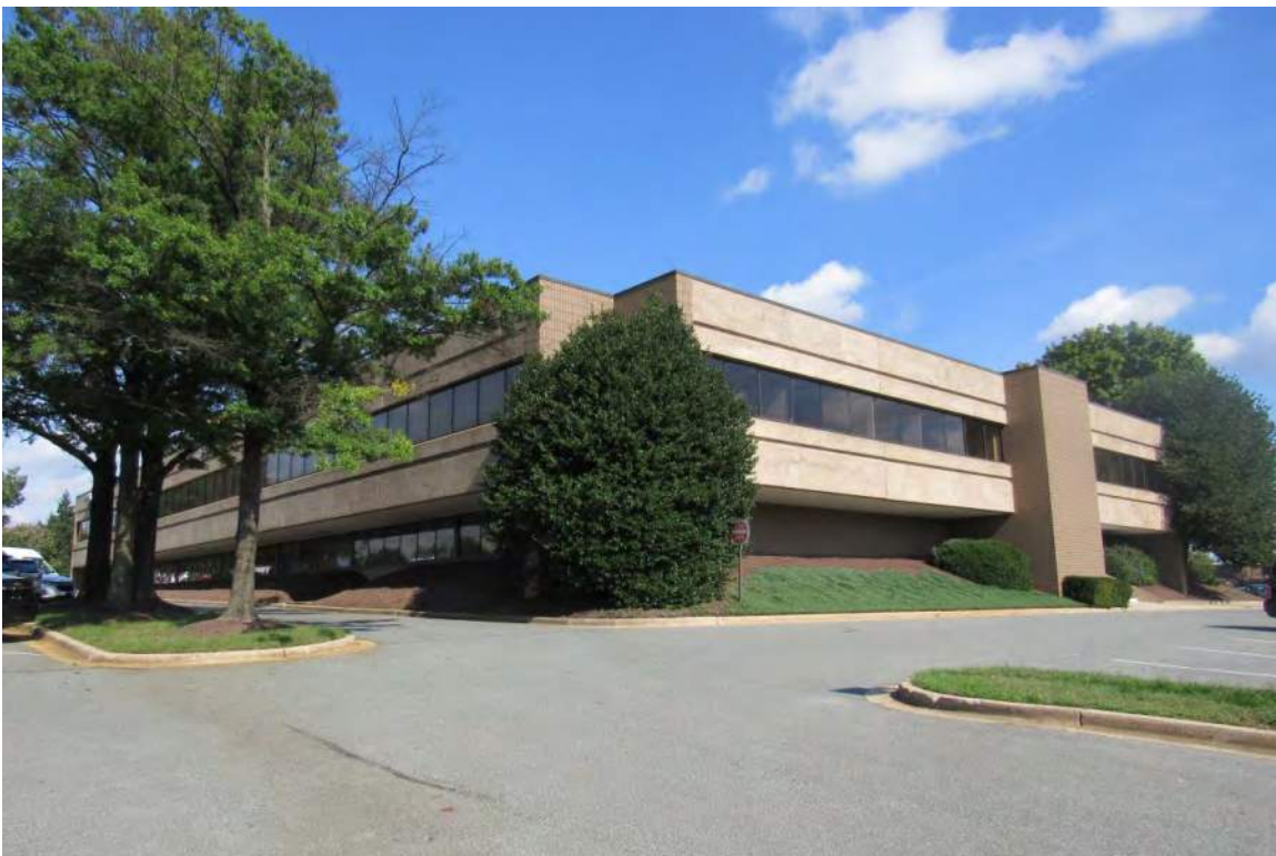
Northwest and southwest facade
