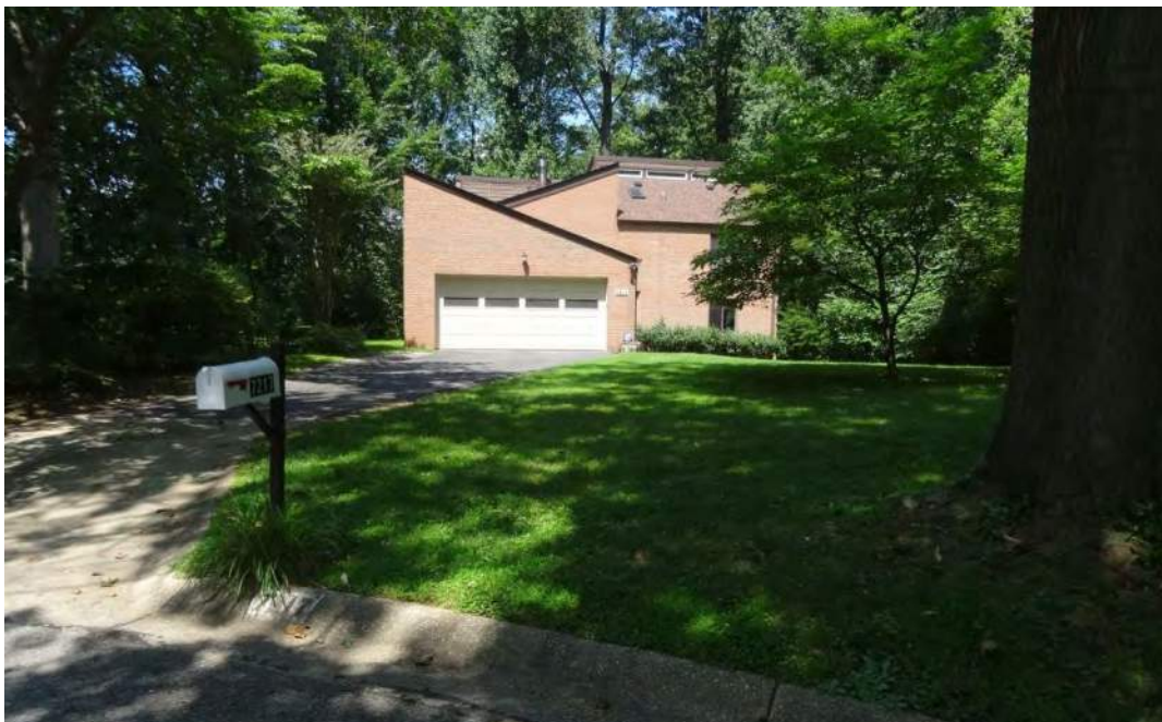
Photo 4 of 7: Southeast elevation of 7217 Grubby Thicket Way.
