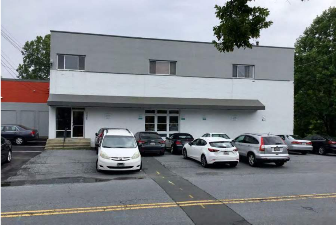
2426 Linden Ave, North Elevation Looking South
