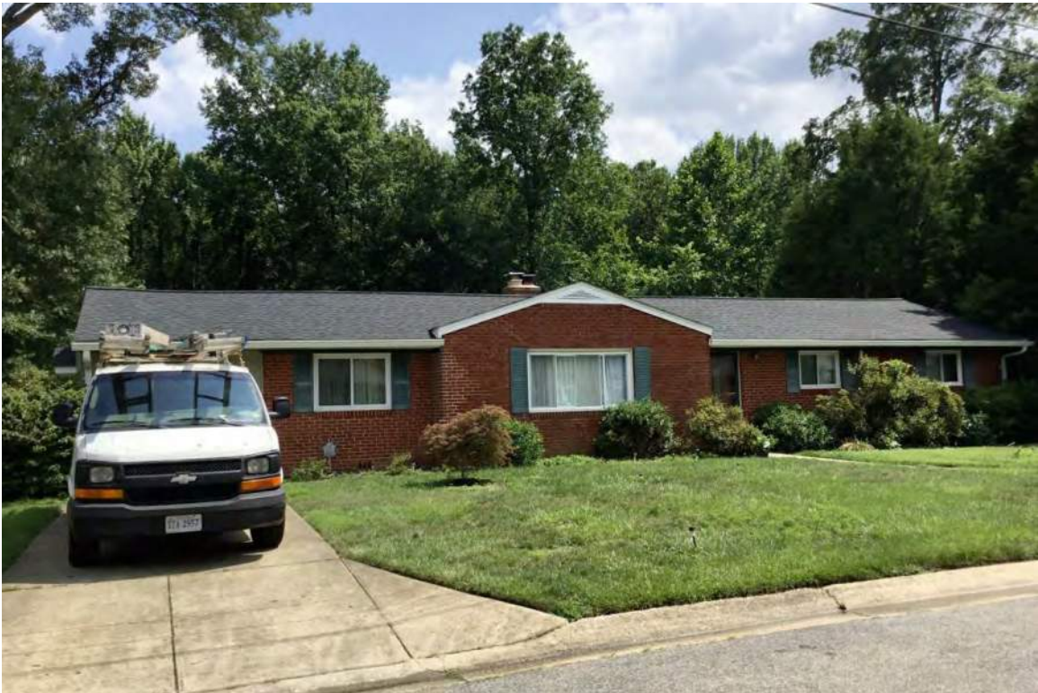
Primary elevation of 5704 Center Drive, looking south.
