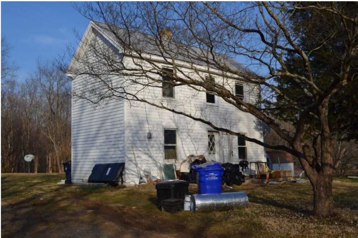
Dwelling, west corner looking northeast
