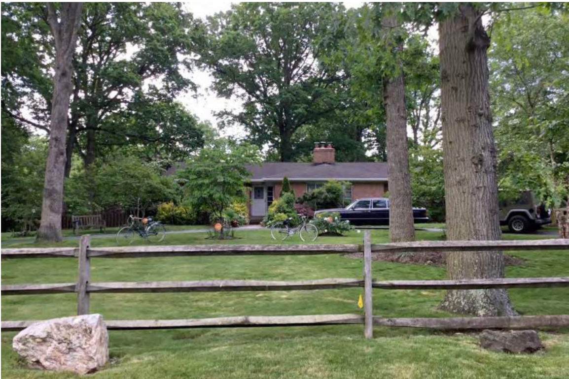
Northwest elevation of 8819 Saunders Lane, looking southeast.
