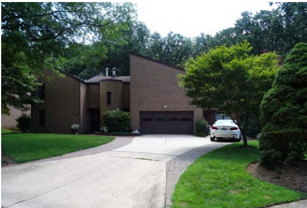
Photo 3 of 7: North elevation of 7220 Grubby Thicket Way.
