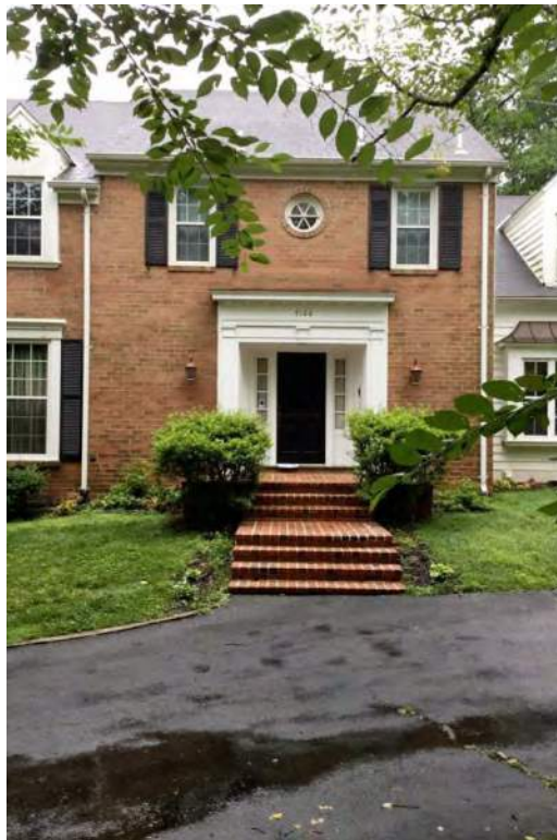
Elevation and entrance detail of 7100 Heatherhill Road, looking southwest.
