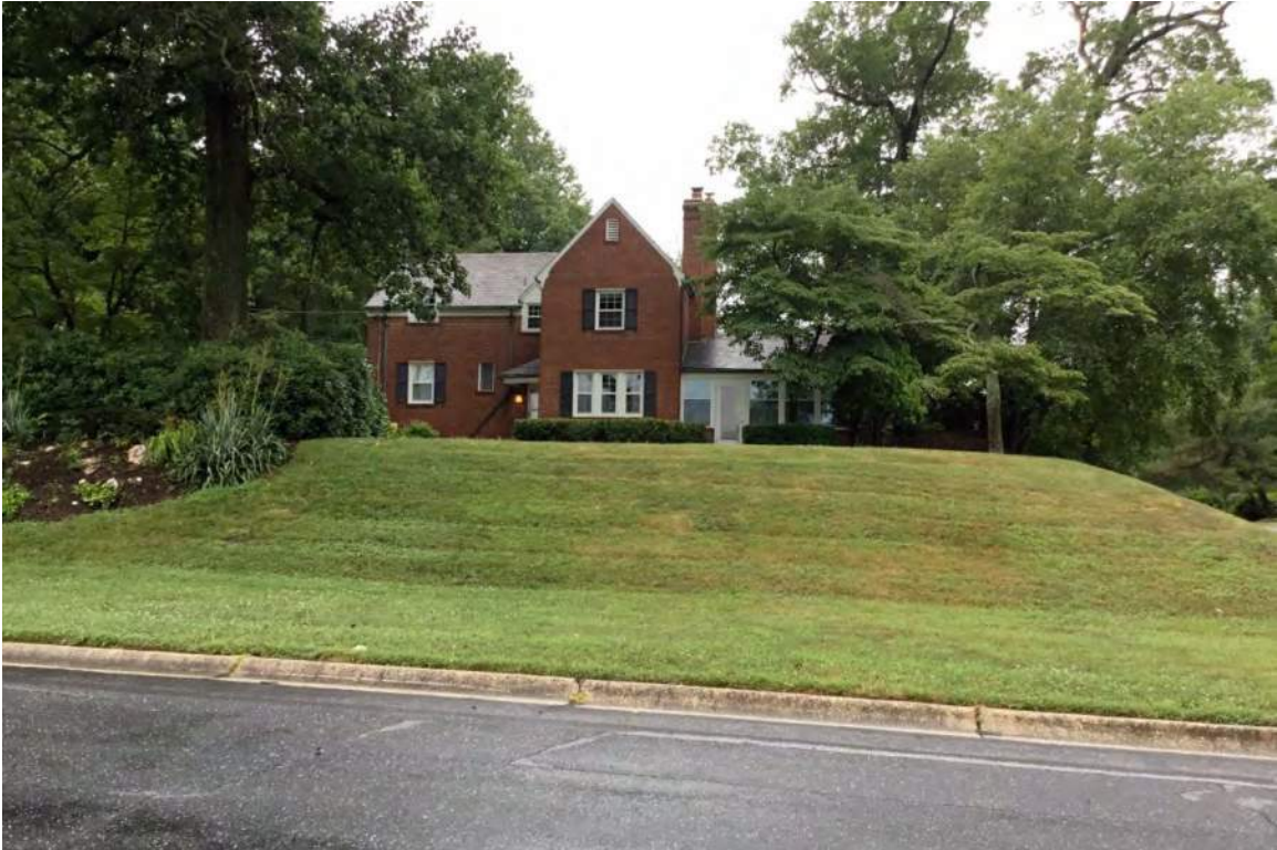
East elevation (façade) of 7124 Greentree Road.
