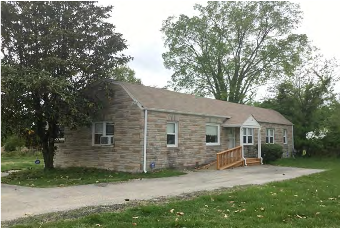
Oblique of 5401 Florist Place, looking northwest.
