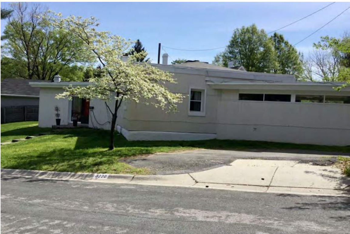
View of 3220 Park View Road, west elevation.
