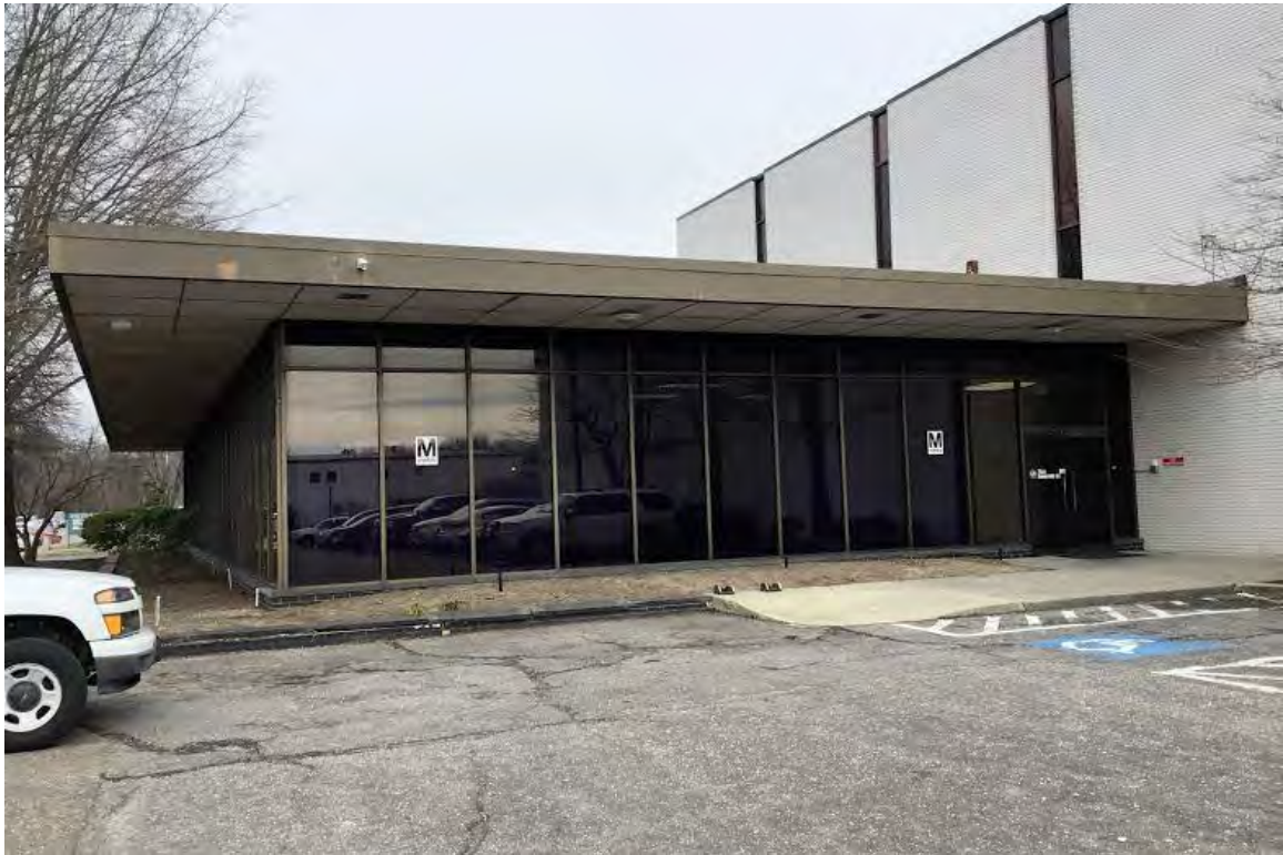
View facing north towards showroom.
