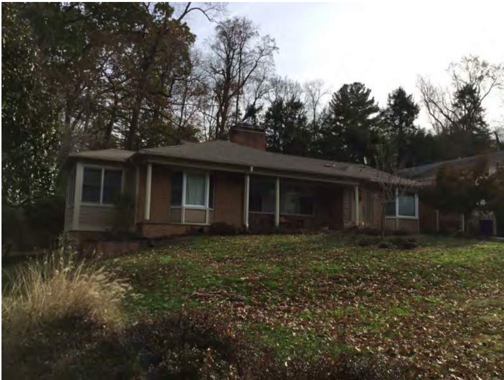
View of east elevation.
