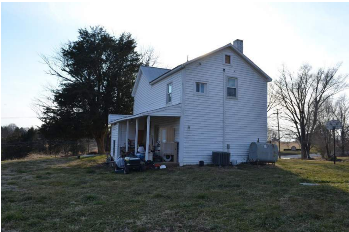
Dwelling, northeast elevation looking southwest
