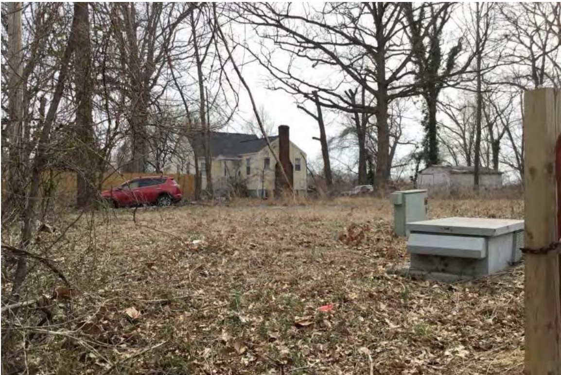
Northwest oblique of 8803 Ardwick Ardmore Road.
