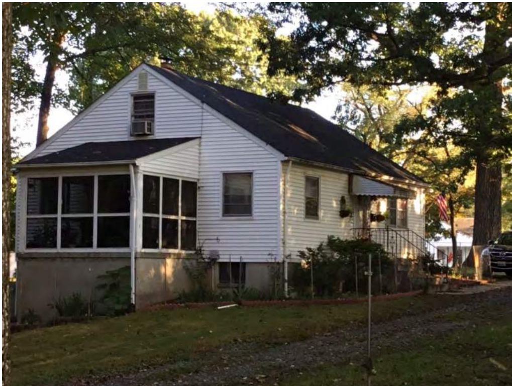
South oblique of dwelling
