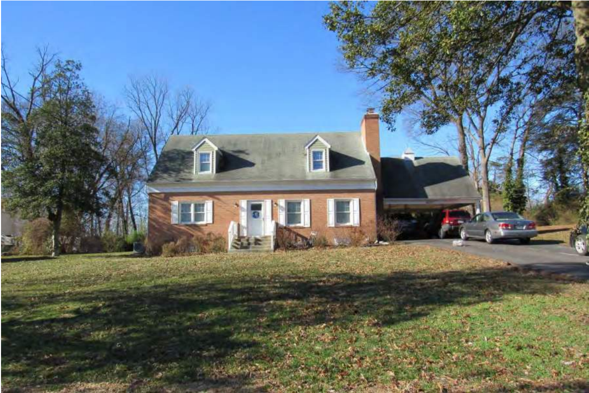
View of 6010 Princess Garden Parkway, looking west.
