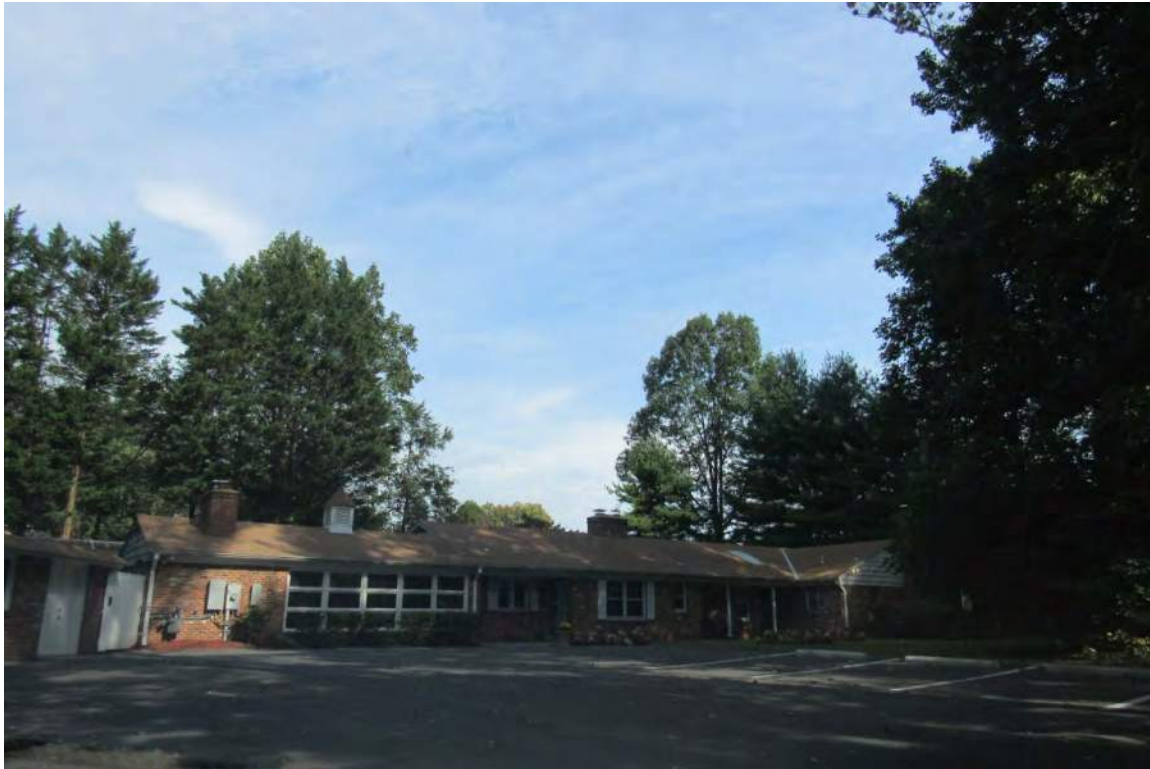
Southeast elevation (façade)
