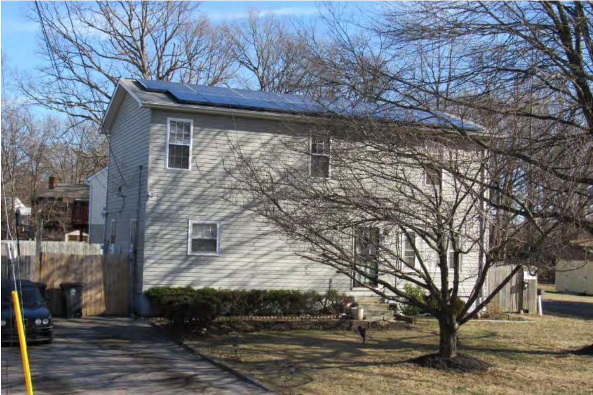
House at 4933 Whitfield Chapel Road, east elevation.
