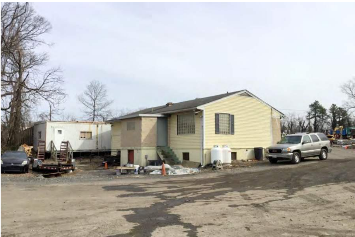
Southwest oblique of 3724 Brightseat Road, looking northeast.
