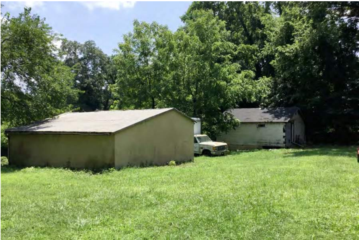
Northeast oblique of machine shed and outbuilding.
