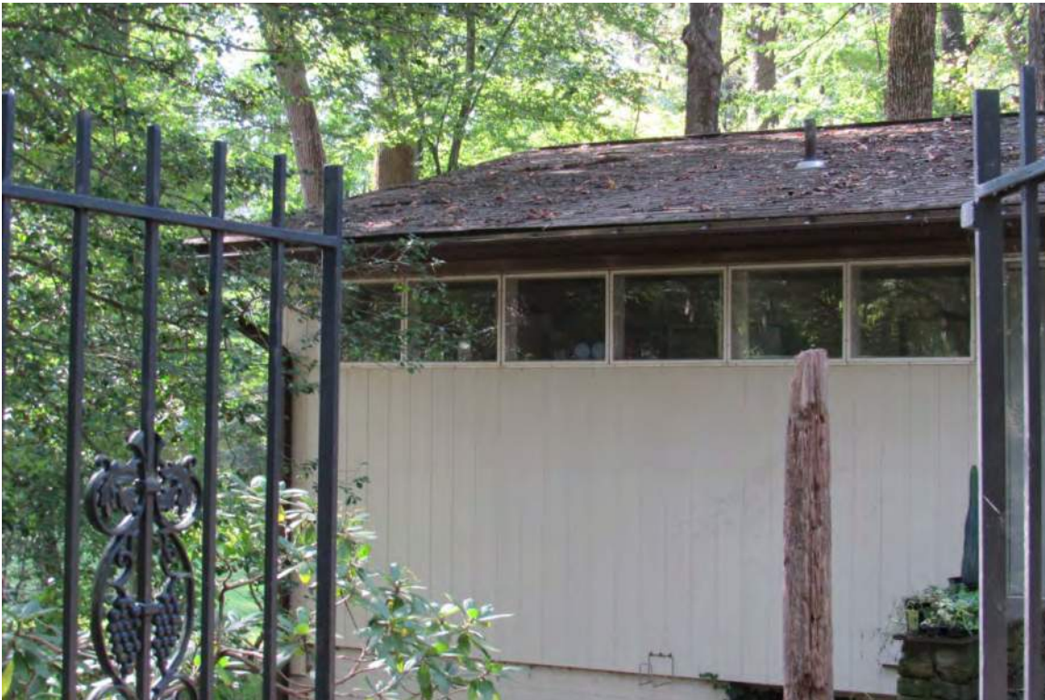
North elevation window detail
