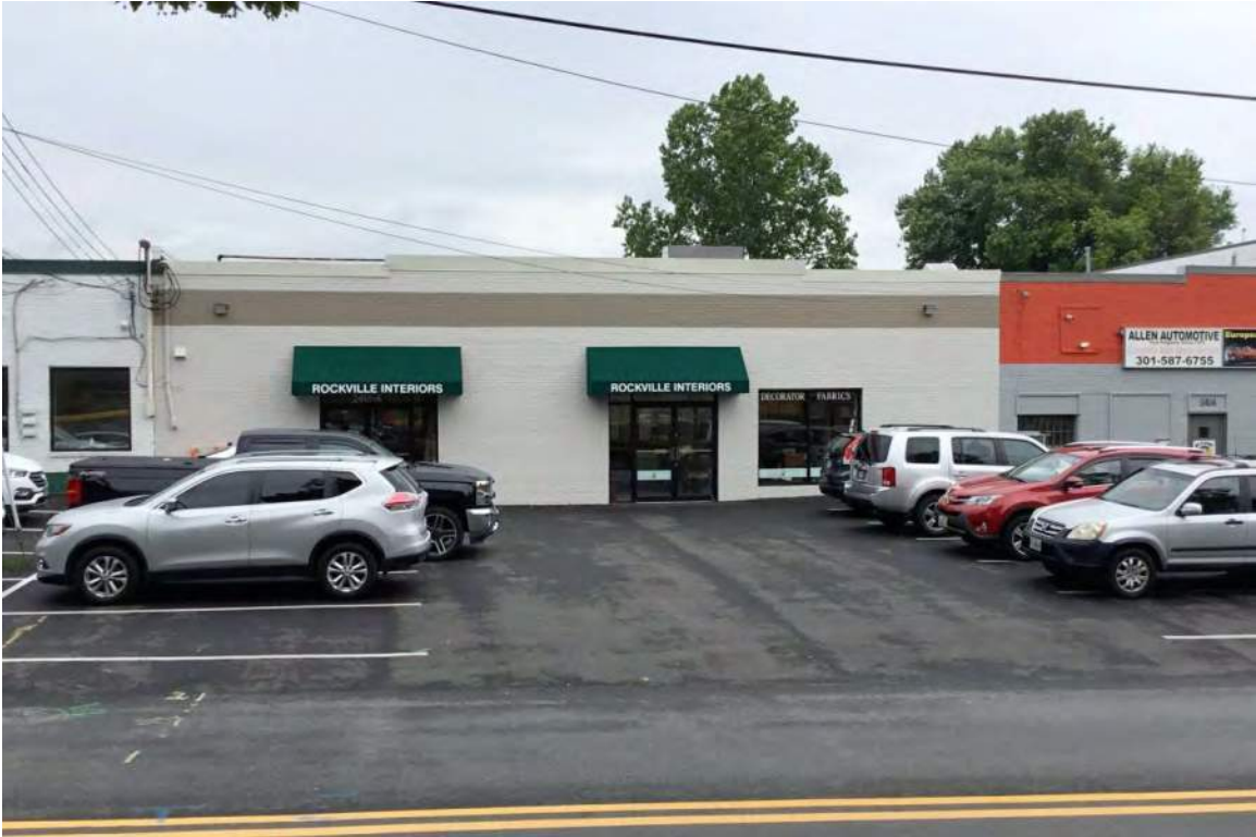
2418 Linden Ave, North Elevation Looking South
