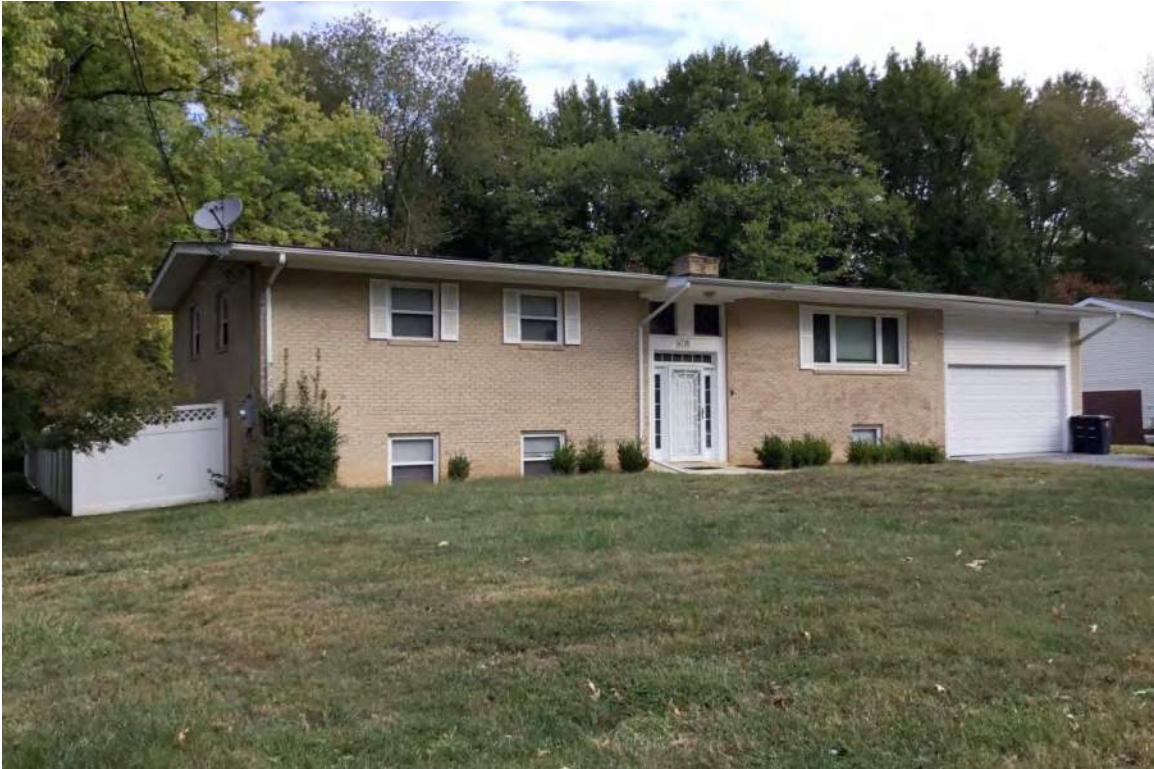
Southwest oblique of 6712 McKeldin Drive.
