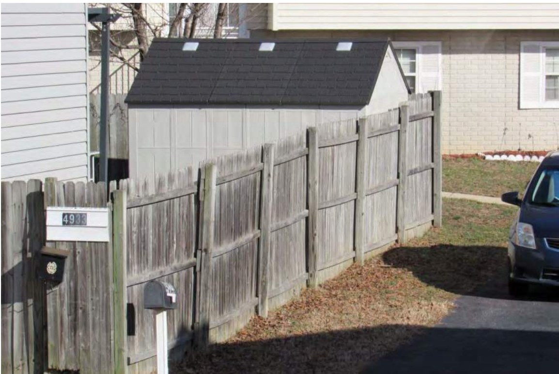
Shed at 4933 Whitfield Chapel Road, east elevation.
