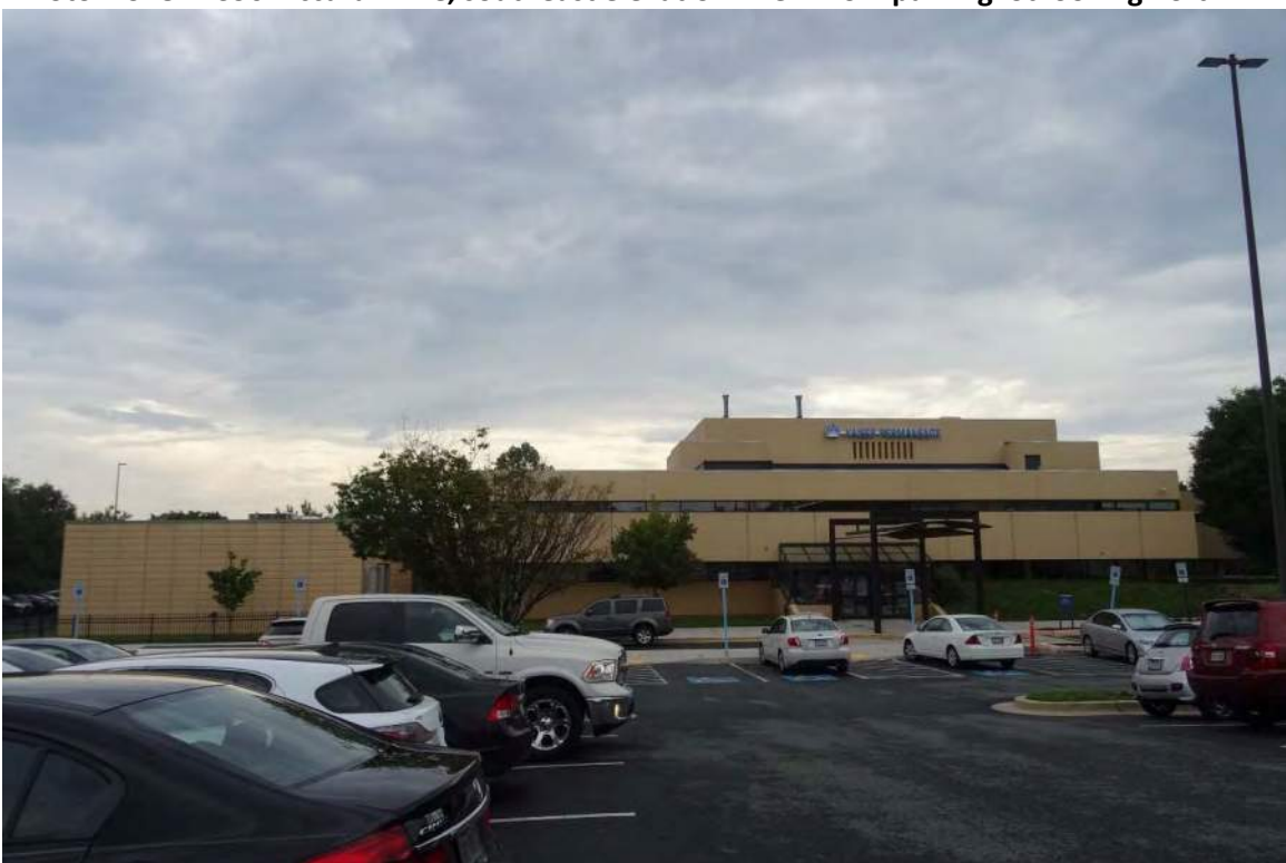
Photo 8 of 8: 1396 Piccard Drive, northeast elevation. View from parking lot looking southwest.
