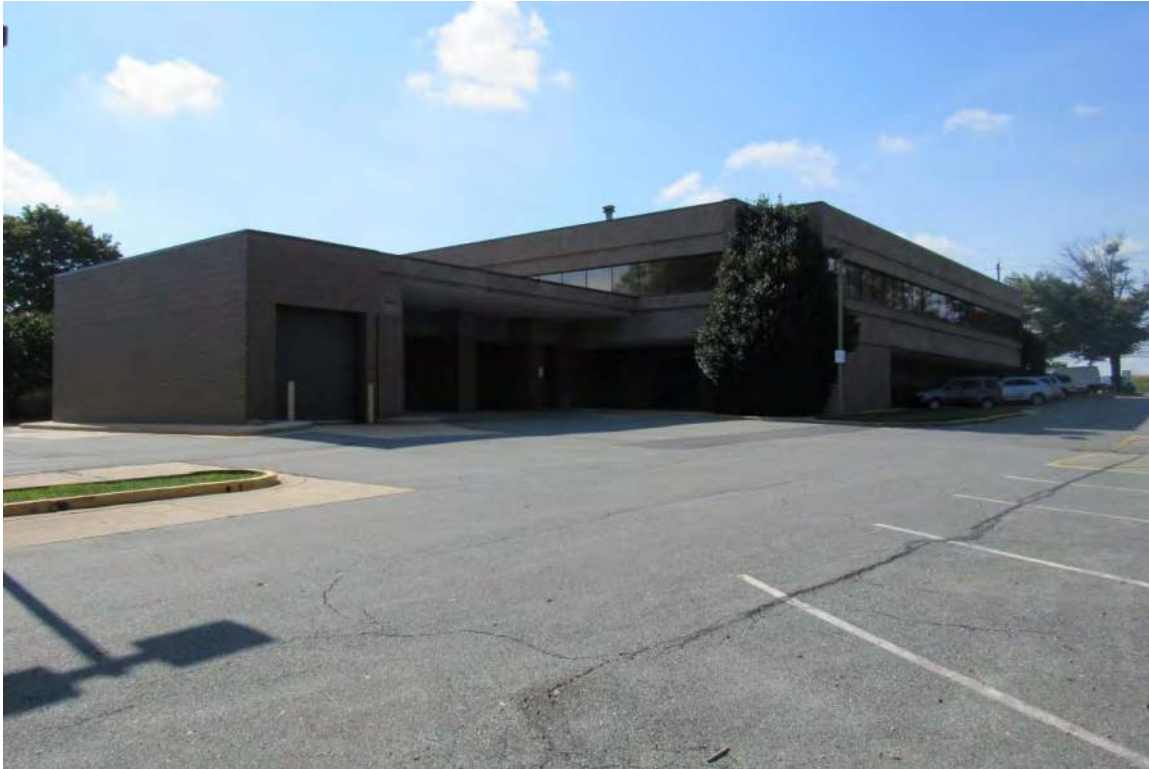
Northeast elevation and service wing at southeast elevation
