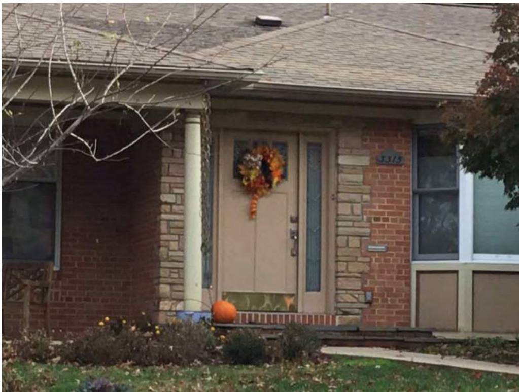
View of front door, looking east.
