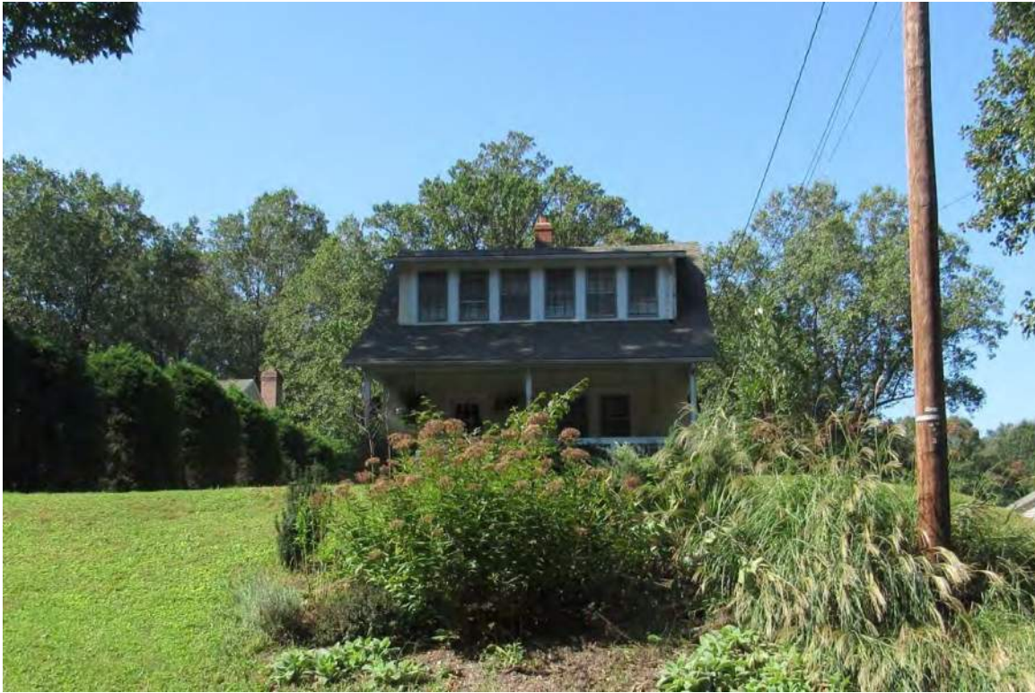
6940 Seven Locks Road, east elevation
