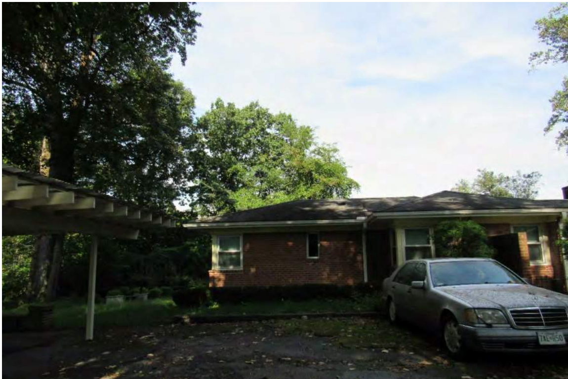
Southeast elevation (façade)
