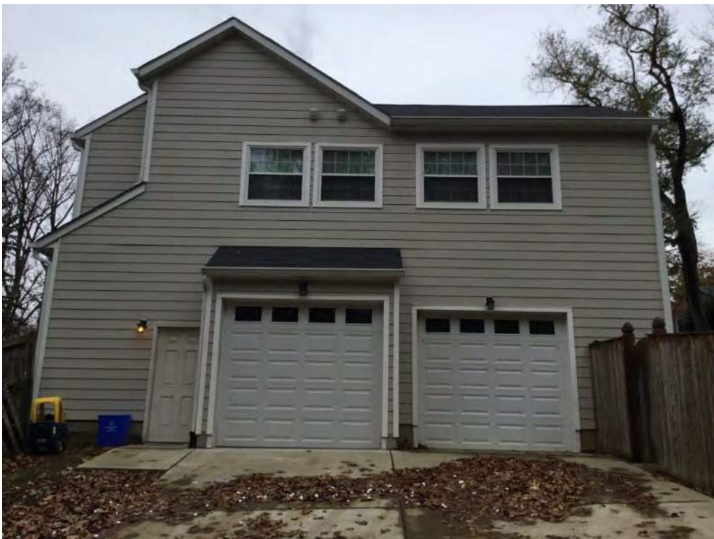
East elevation and addition.
