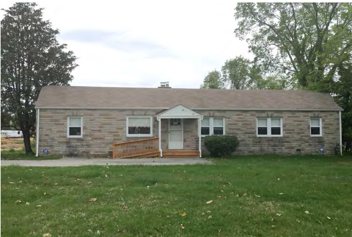
Façade of 5401 Florist Place, looking southwest.
