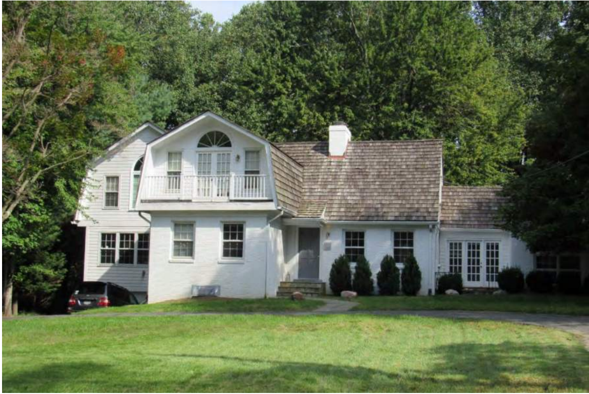
Southwest elevation (façade)
