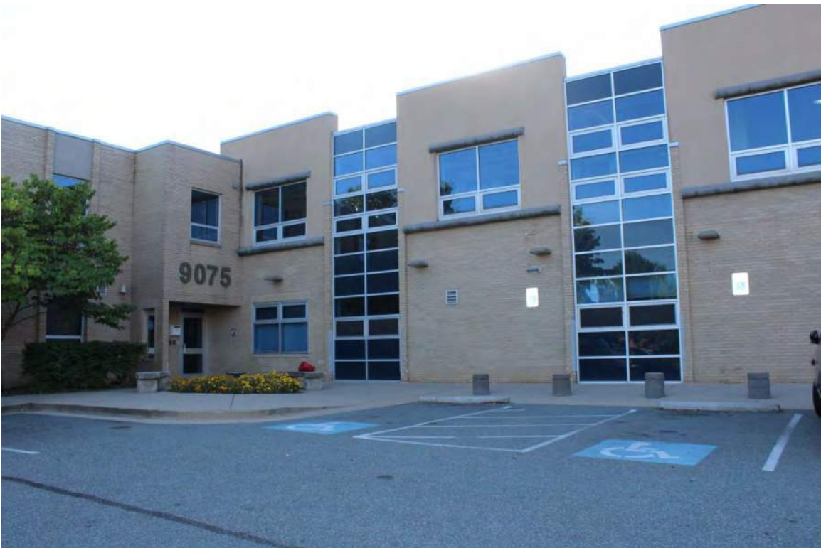
Entrance and window detail at west elevation
