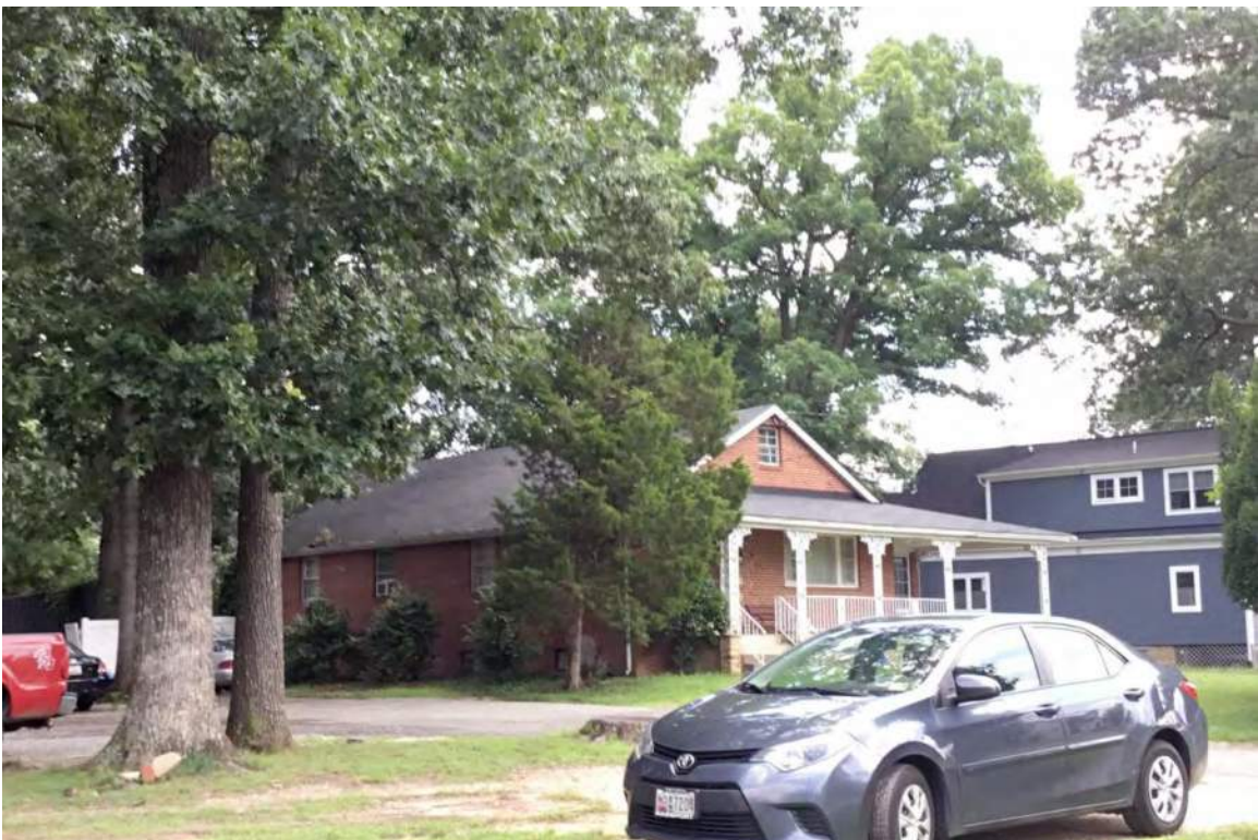
East oblique of 5502 Old Branch Avenue.
