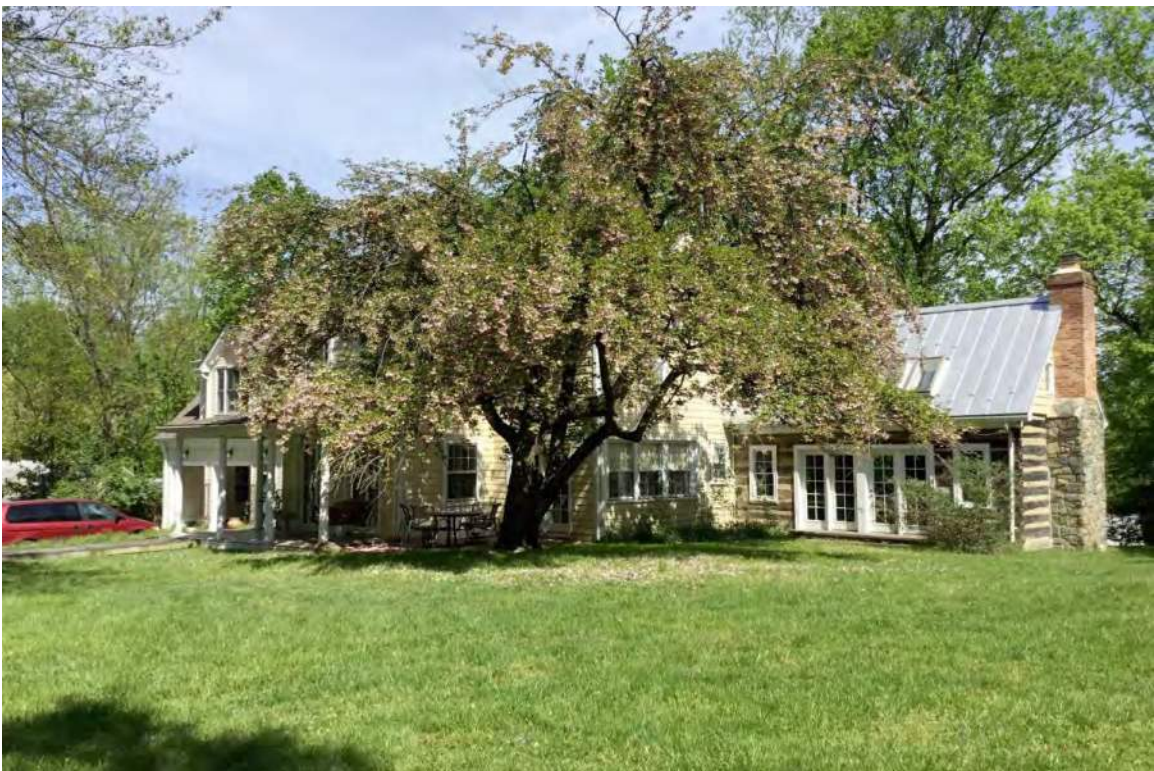
Oblique of 9017 Spring Hill Lane, looking northwest.
