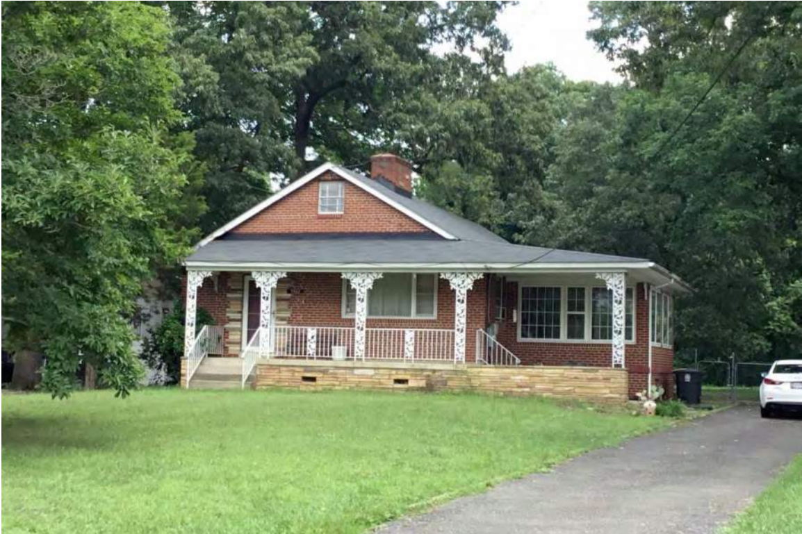
Southwest elevation of 5502 Old Branch Avenue.
