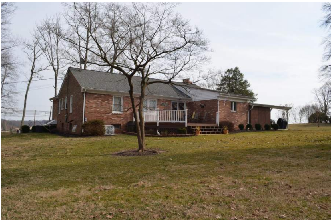
Dwelling, northwest elevation looking east
