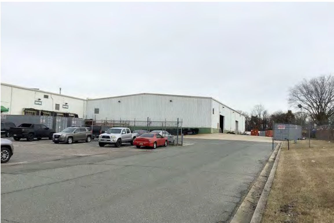
View facing east towards southern pole building at 3900 Penn Belt Place.
