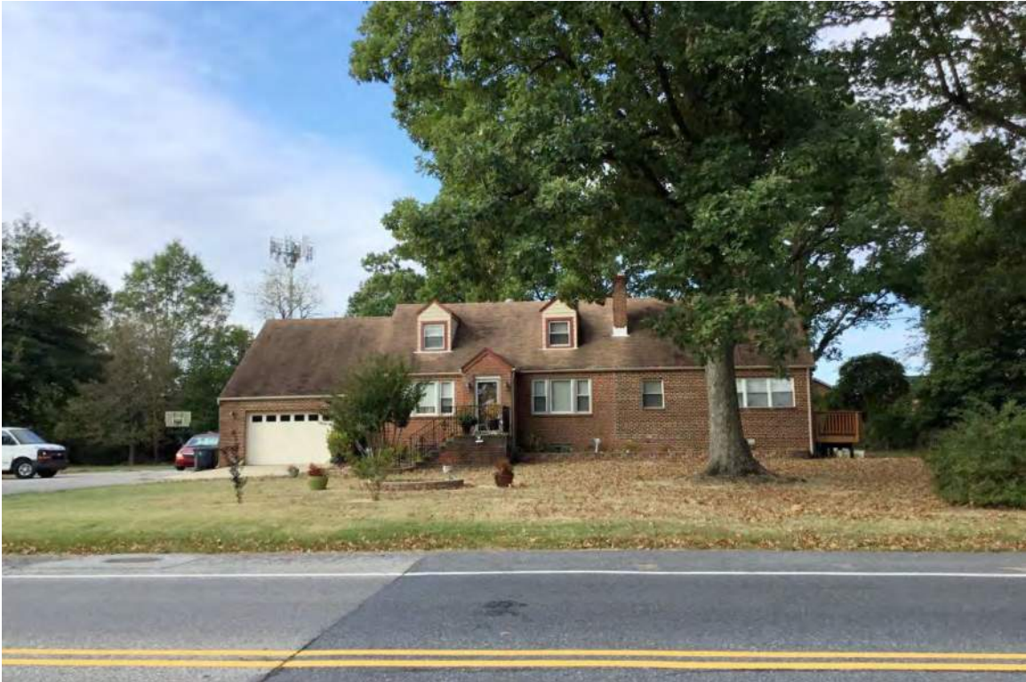
Northeast elevation of 6001 Auth Road.
