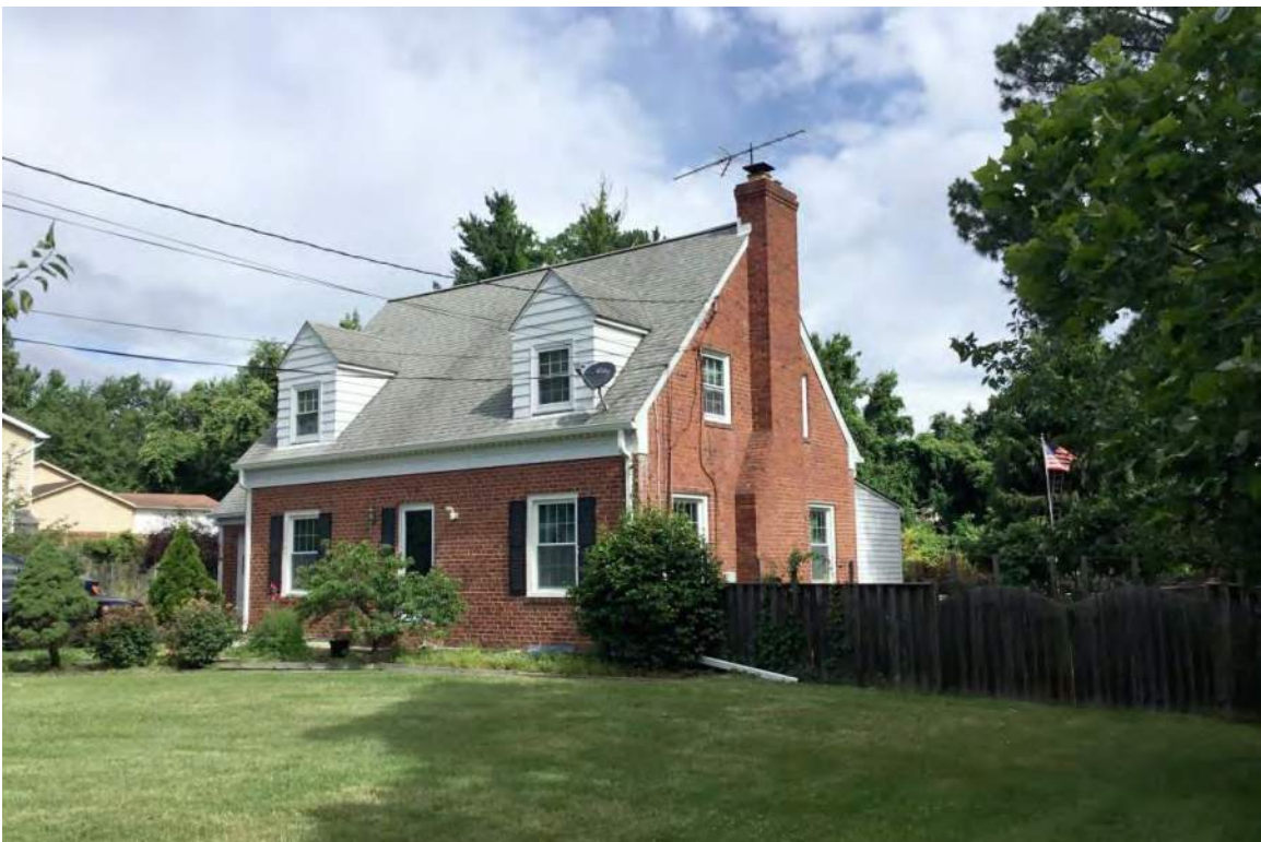
South facade and east elevation
