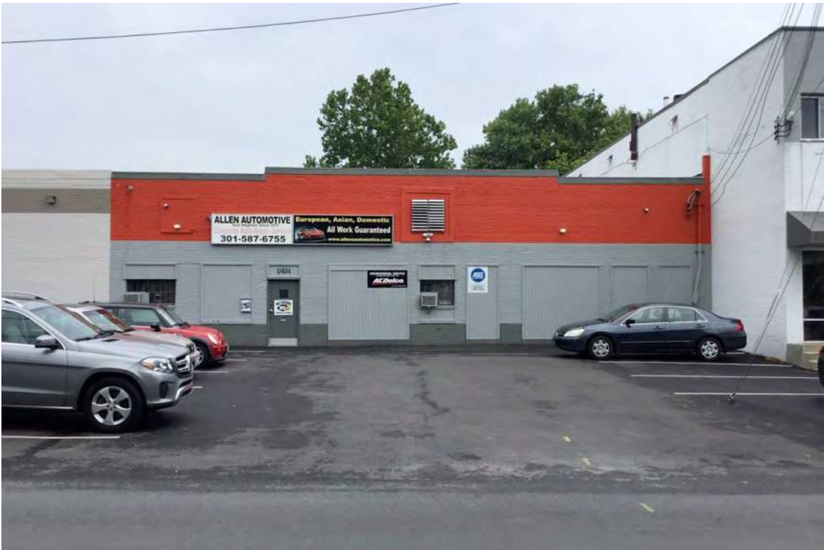
2424 Linden Ave, North Elevation Looking South
