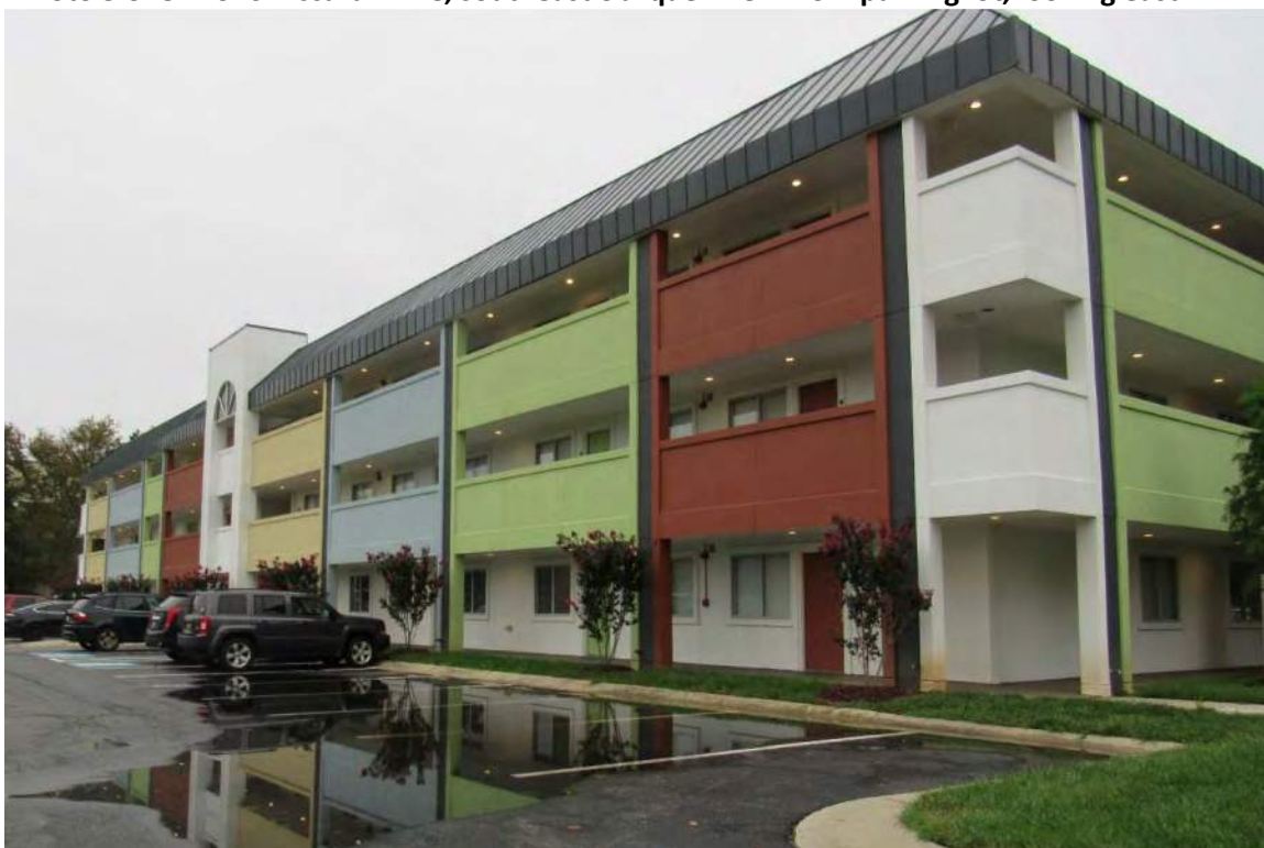
Photo 6 of 8: 1380 Piccard Drive, northeast oblique. View from parking lot, looking northeast.
