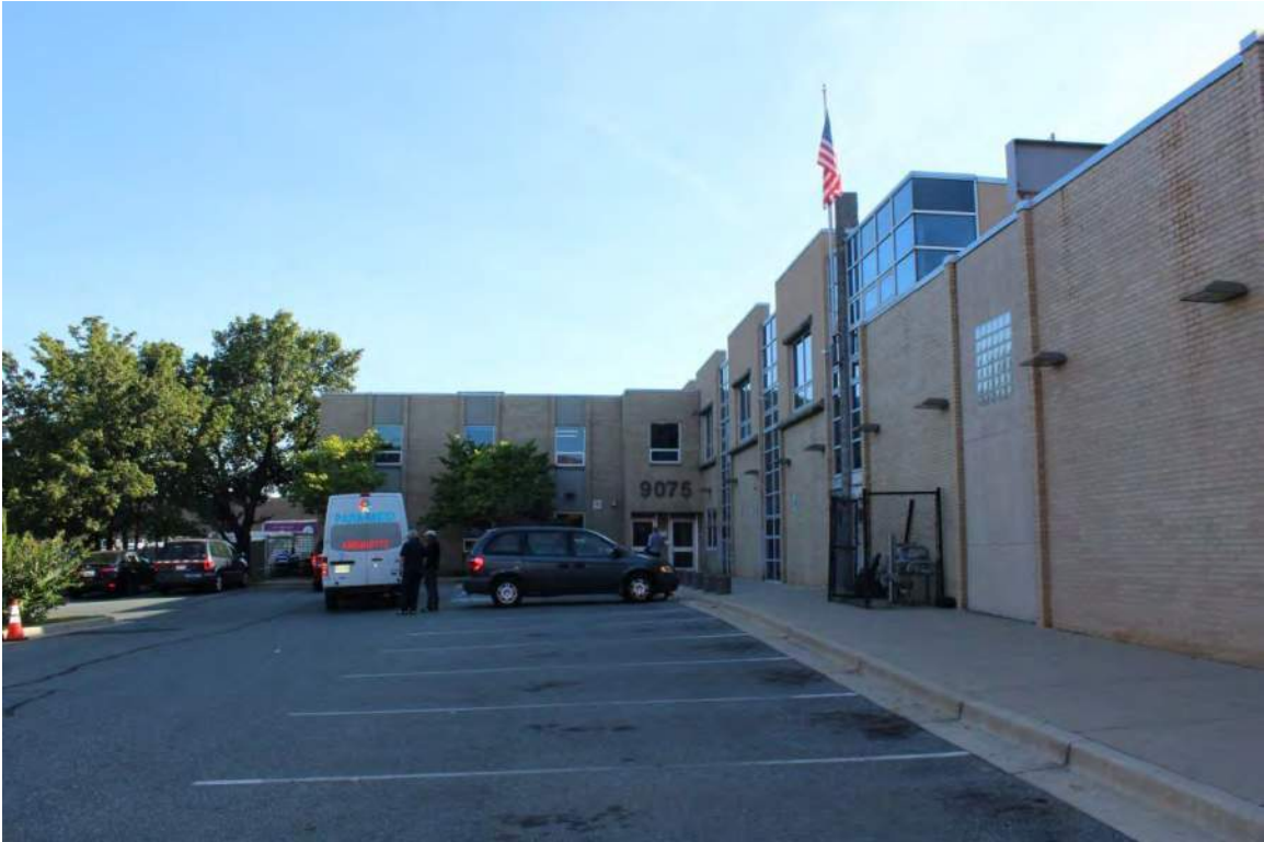
View south along east elevation to south ell
