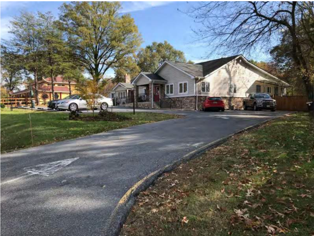
Oblique showing north facade and west elevation
