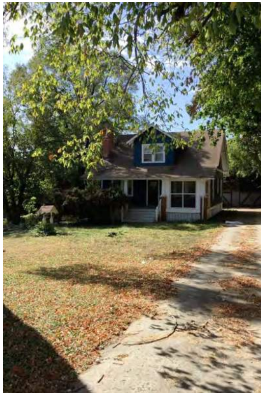
223 University Boulevard East, East Elevation Looking West
