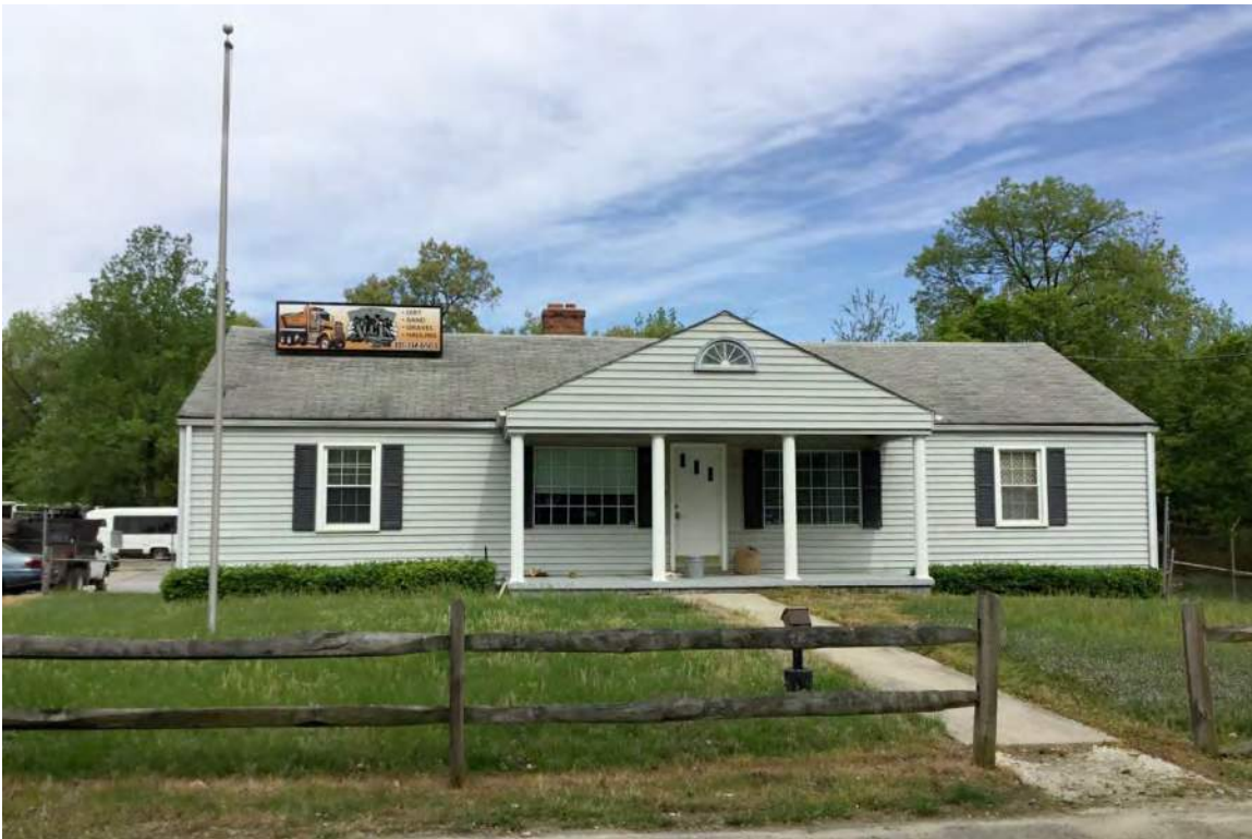
Southeast elevation (façade) of 4704 Medley Drive, looking northwest.
