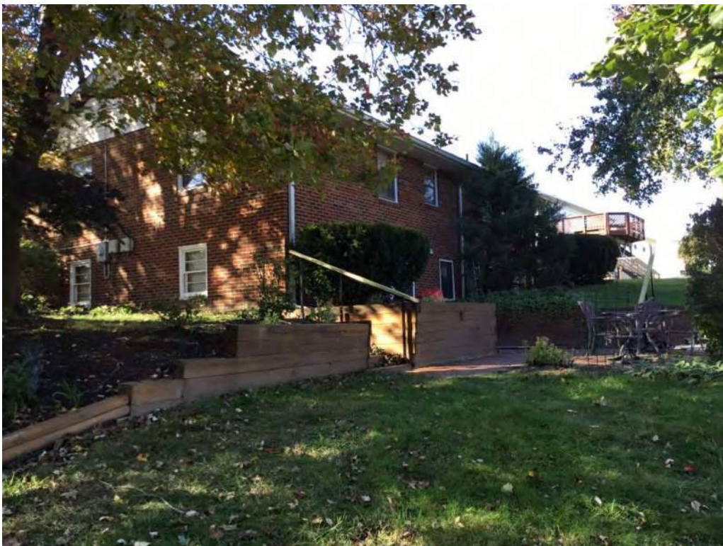
Southeast oblique of 9907 51st Avenue, looking northwest.
