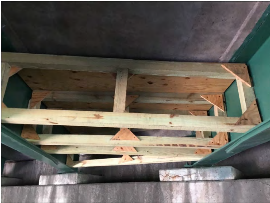
Photo 24: Greenbelt Road Outer Loop (141015) - Wooden braces obscure view of and access to the northwest abutment wall.
