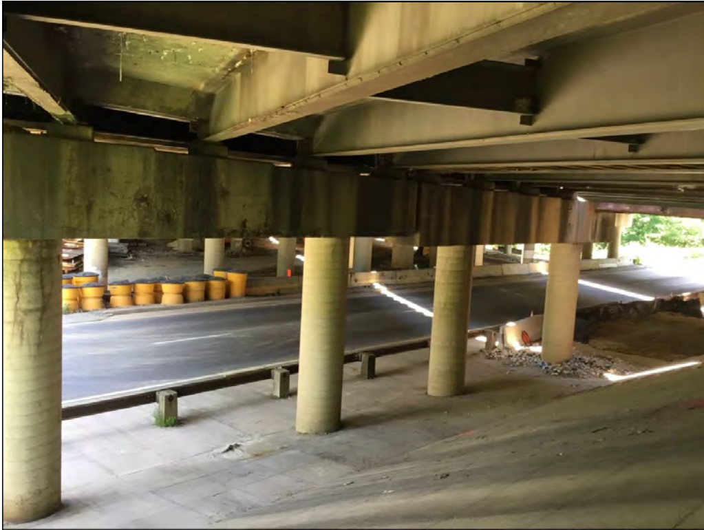
Photo 31: Suitland Parkway Outer Loop (160015) - Looking southwest at piers. Gaps between pier caps may provide roosting locations for bats.
