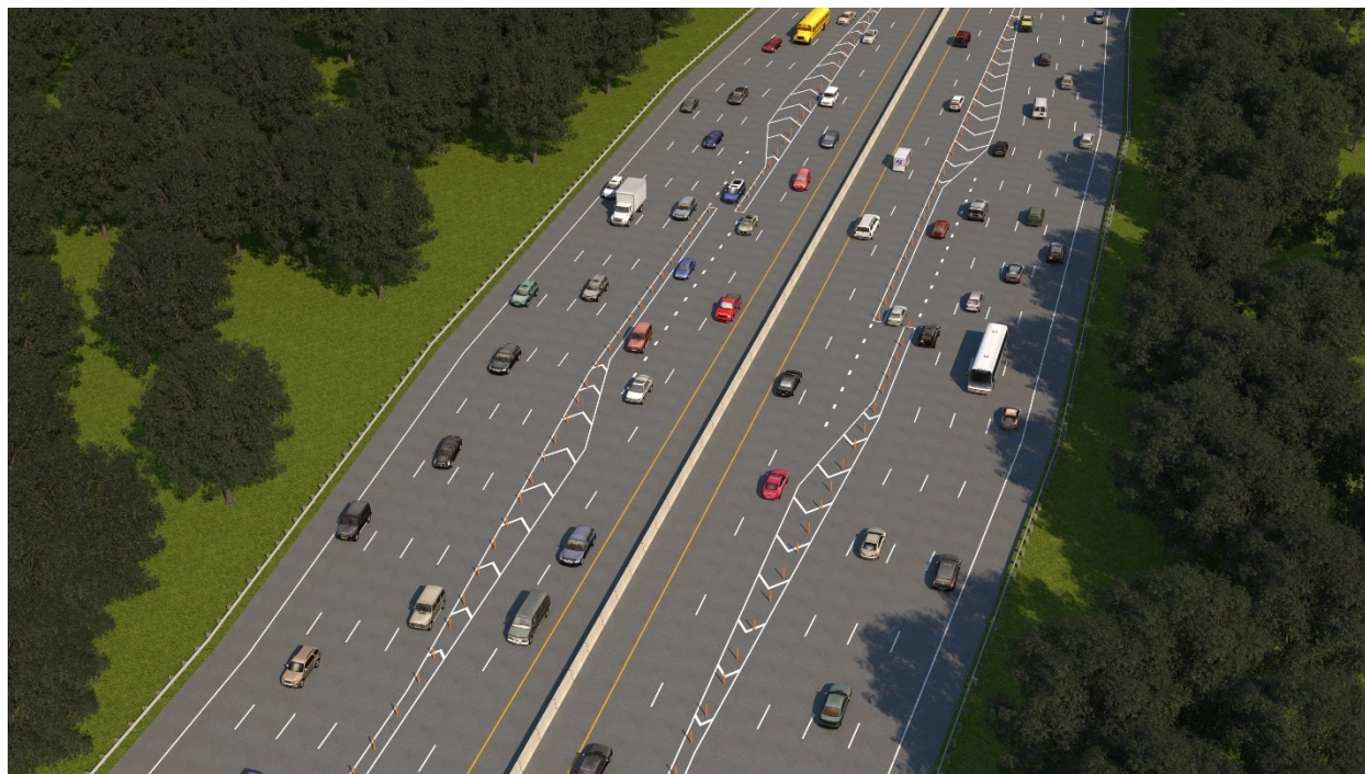
Figure 2-13: Example At-Grade Access Slip Ramp Configuration
