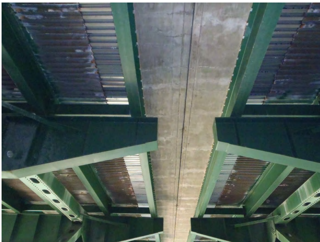
Photo 80: Northwest Branch (137010) – Looking at gap in deck between inner and outer loops
