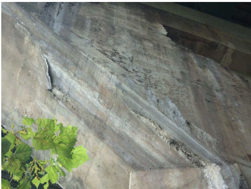
Photo 4: American Legion Bridge North (100010) – Looking at cracks in pier
