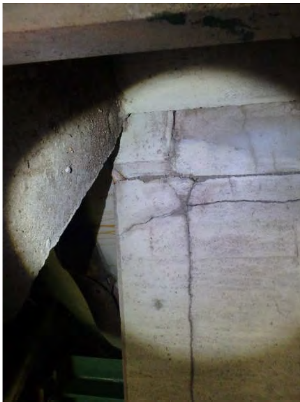
Photo 27: Seven Locks Road (106010) – looking at cracks in concrete support between inner and outer loops
