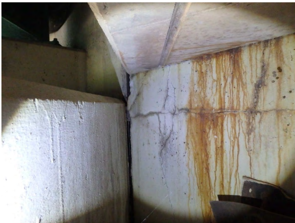
Photo 32: Cabin John Parkway (108010) – Looking at vertical crevice in north abutment
