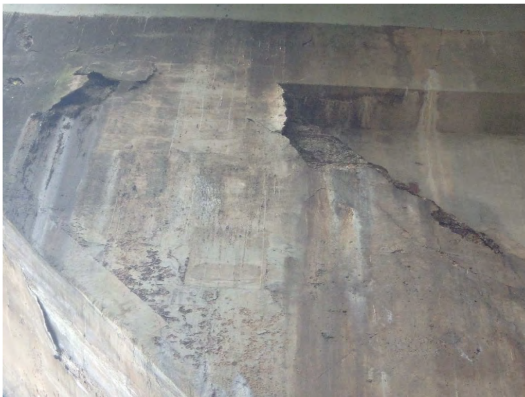
Photo 3: American Legion Bridge North (100010) – Looking at cracks in pier
