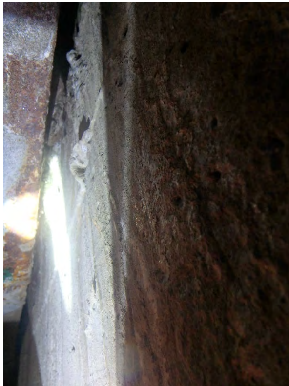
Photo 58: Cedar Lane (122010) – Looking at crack between abutment and deck on east abutment
