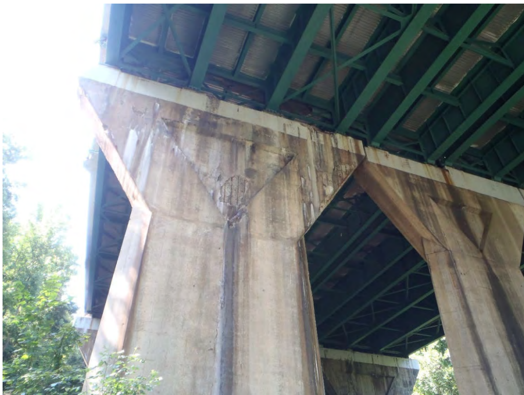
Photo 9: American Legion Bridge South (100010) – Looking at cracks in piers
