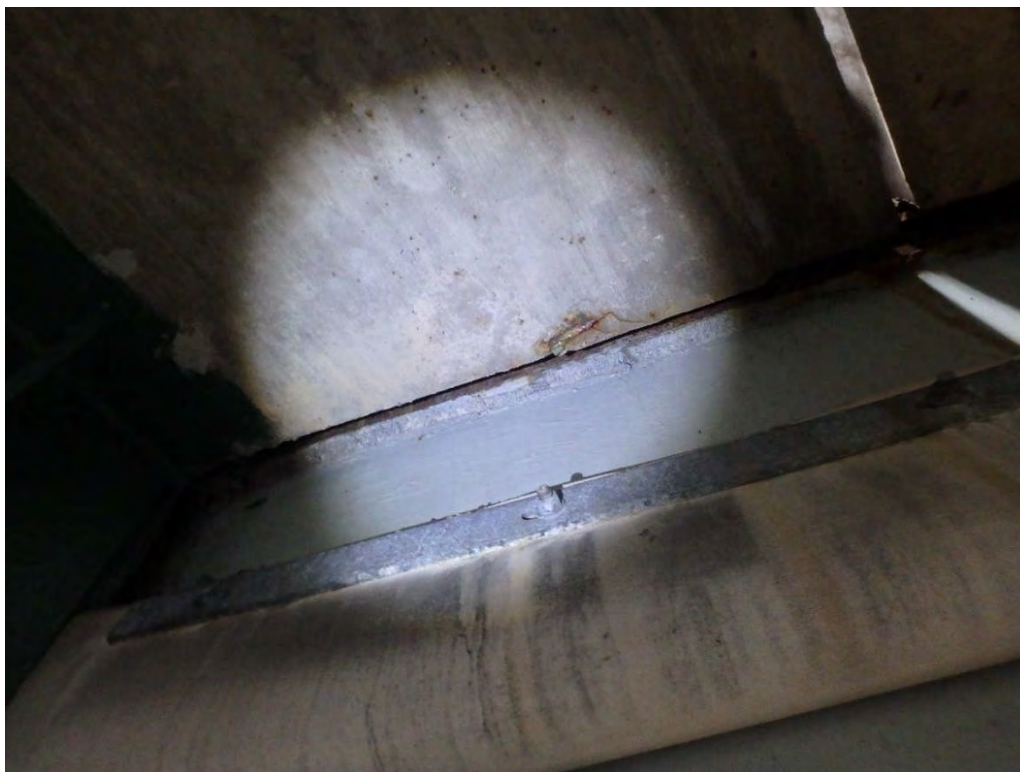
Photo 47: River Road (110010) – Looking at crack along west abutment
