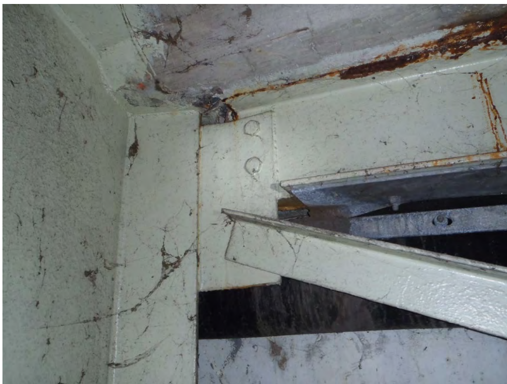
Photo72: Rock Creek/Stoney Brook Drive (126010) – Looking at corner gap on abutment wall
