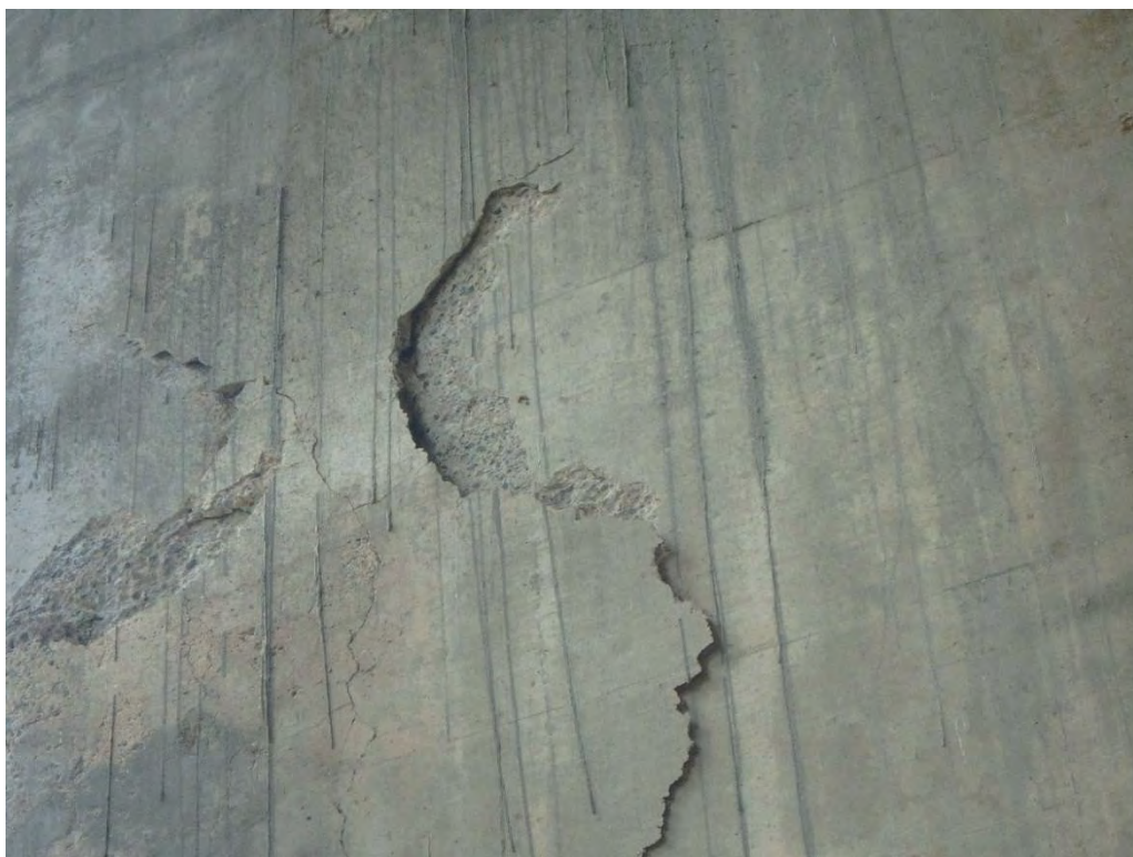
Photo 2: American Legion Bridge North (100010) – Looking at cracks in pier
