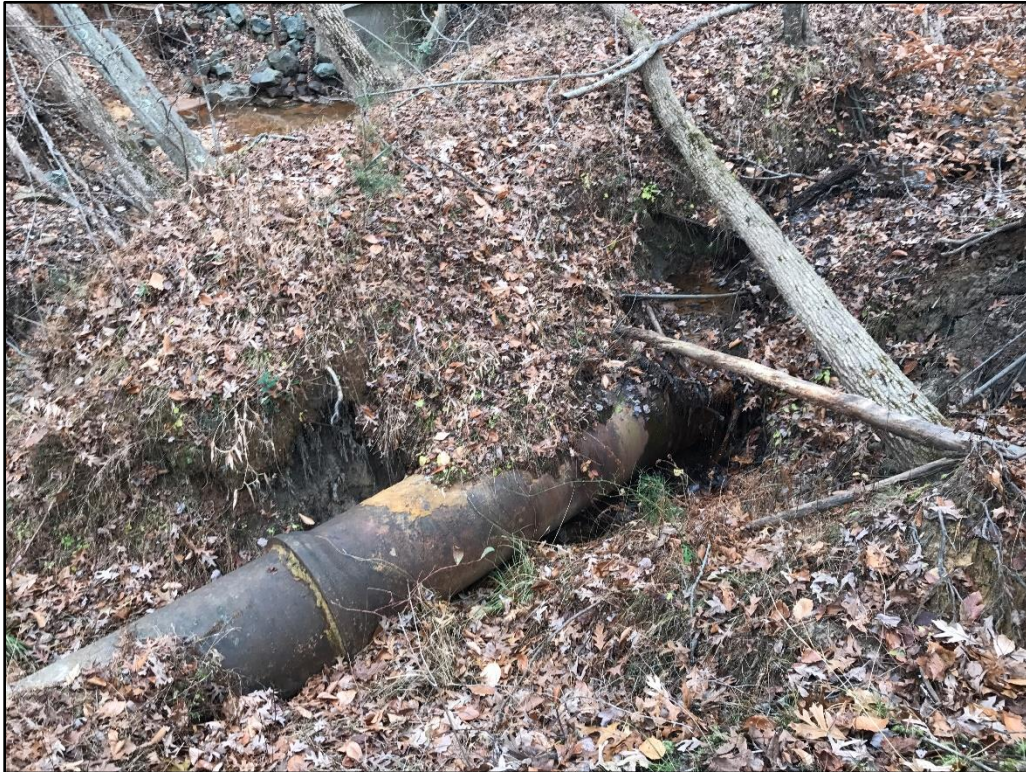
Figure 81. Cast iron pipe running through trench in Area S-26, facing southwest
