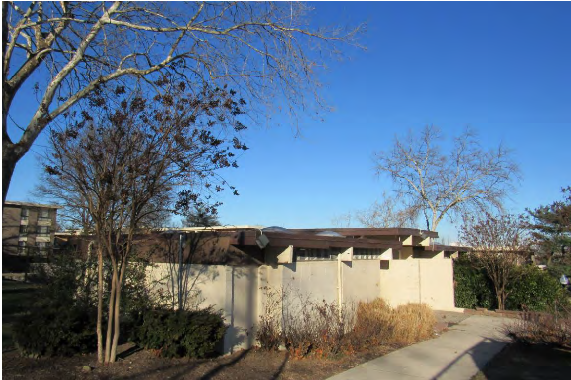
View of pool changing facility, facing northeast.
