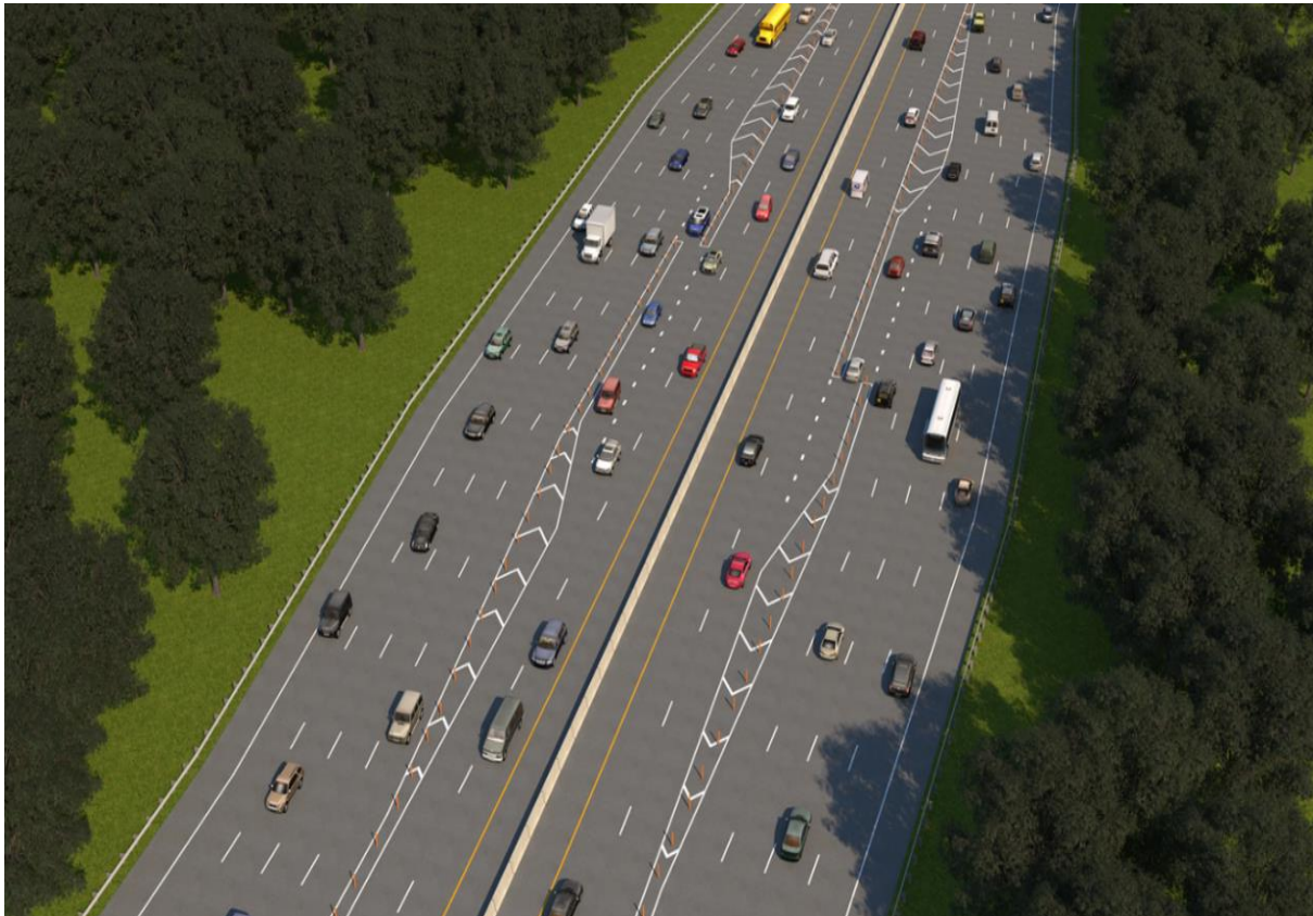
Figure 22: At-Grade Access Illustration
