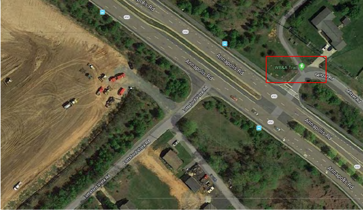
Image 3, WB&A trailhead at site of construction
