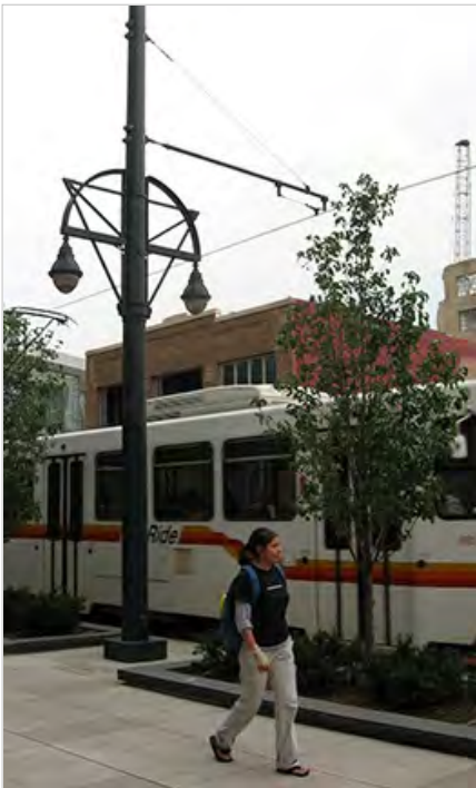
Figure 6-14. Fixed-Termination Single Contact Wire Sharing a Pole with Street Lights
