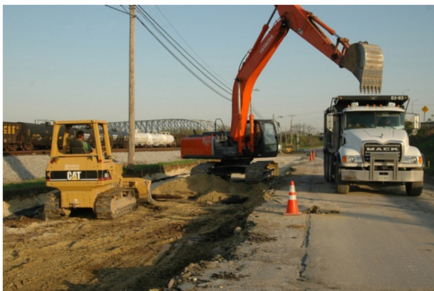
Figure 5-4. Example of Road Cut for Track Installation
