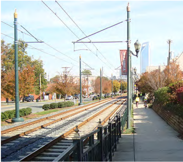
Figure 6-14. Fixed-Termination Single Contact Wire Sharing a Pole with Street Lights
