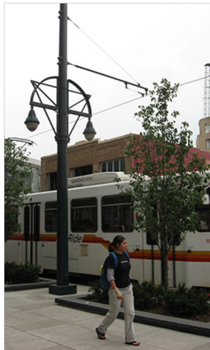
Figure 2-19. Fixed-Termination Single Contact Wire Sharing a Pole with Street Lights
