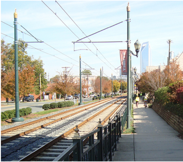
Figure 2-18. Auto Tensioned Catenary System
