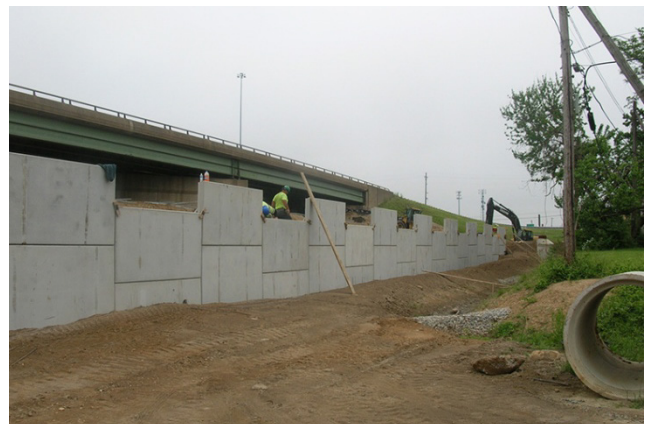
Figure 5-5. MSE Retaining Wall Construction
